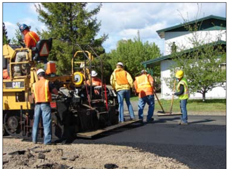
Above is Instructor Roy Hill giving an entry level apprentice pointers on asphalt rolling while another student is sealing a joint for the paving project.
