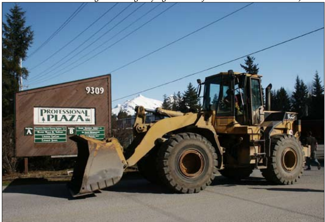
Paving Glacier Highway right outside of District 8 Local 302 Hall in Juneau
