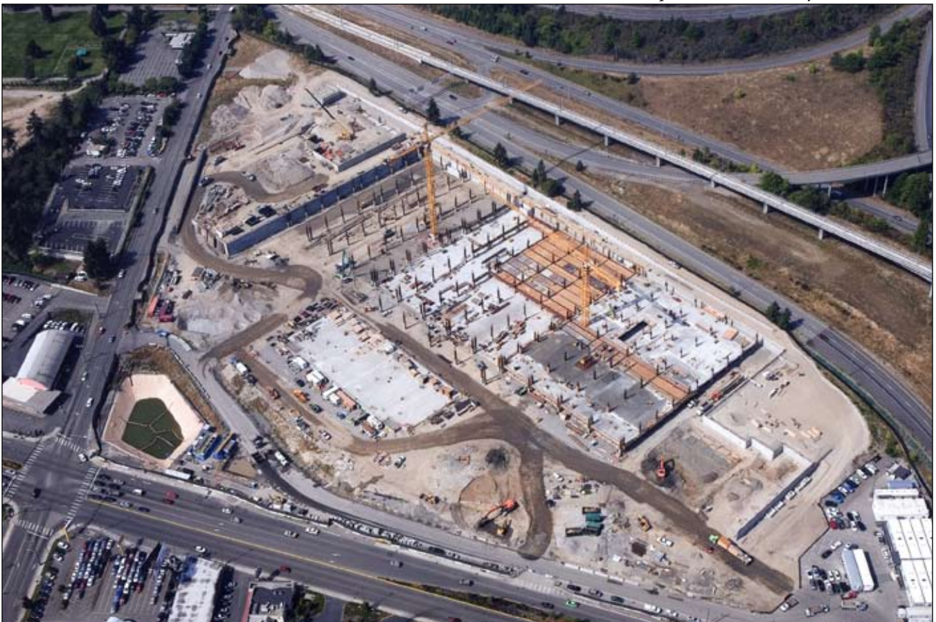
Airport Rental Car Facility Construction Site
