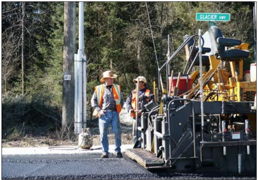
Secon paving project in Juneau
