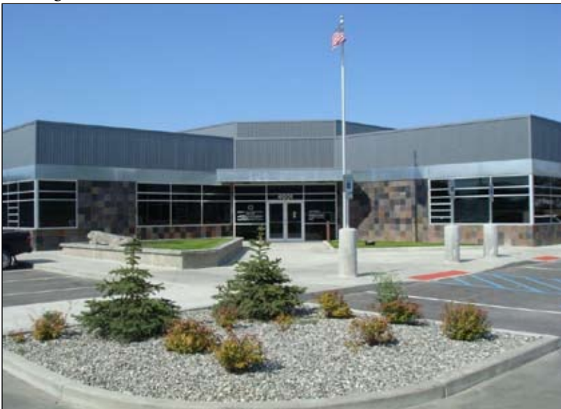
Anchorage Hall Finished
