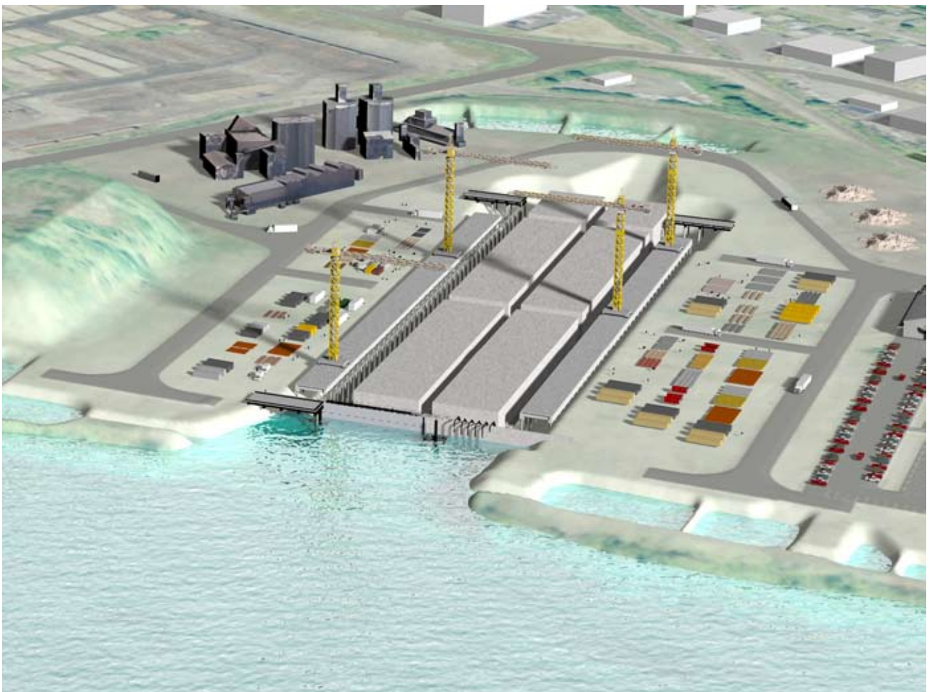
Concrete pontoons for the state Route 520 floating bridge will be assembled in a giant casting basin at a proposed 55-acre site in Aberdeen. The site will also have offices, a rail spur, assembly areas and a concrete batch plant, shown in the upper left.
