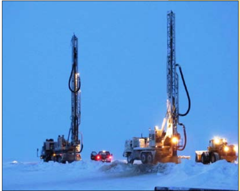
The two drillers are from a recent pipeline class that was held in Prudhoe Bay, Alaska.
