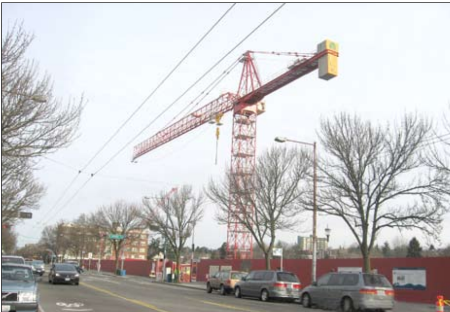
Kroll Tower Crane in Capitol Hill
