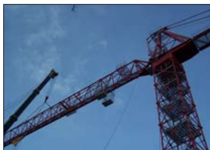
The Kroll 1800 crane at the Sound Transit Link in Capitol Hill
