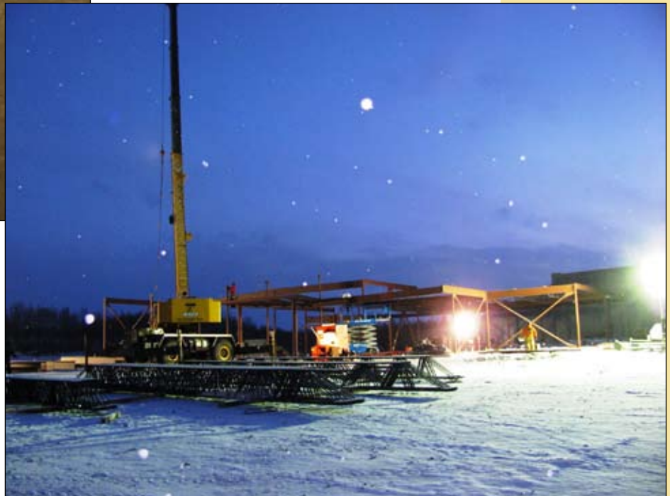
Hanging steel for new Alaska Training Center classroom
