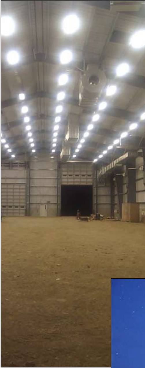
Indoor Arena New Alaska Training Center
