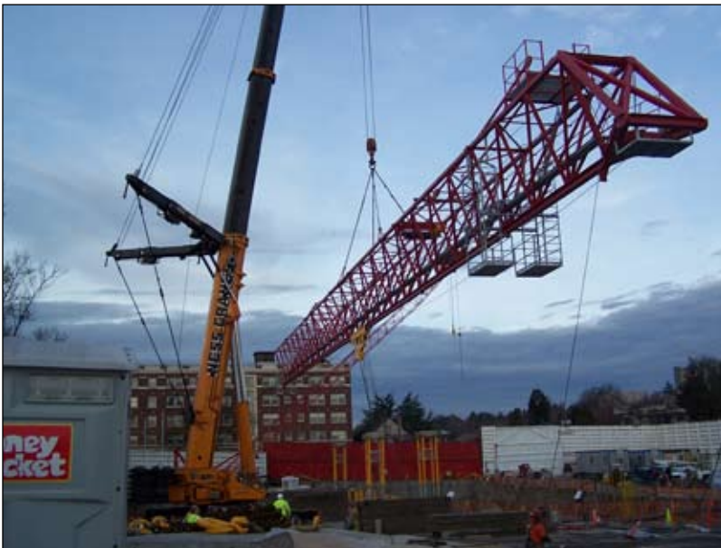
The Kroll 1800 is the largest capacity crane in the United States. It can pick up 32,000lbs. at the tip.
