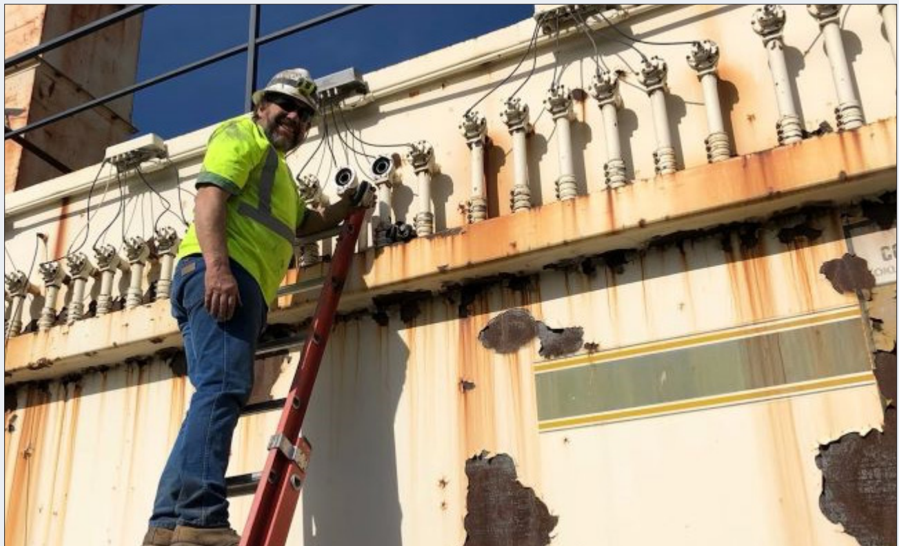
Below: Ray Porter of Granite Construction performing Asphalt Plant Maintenance.
