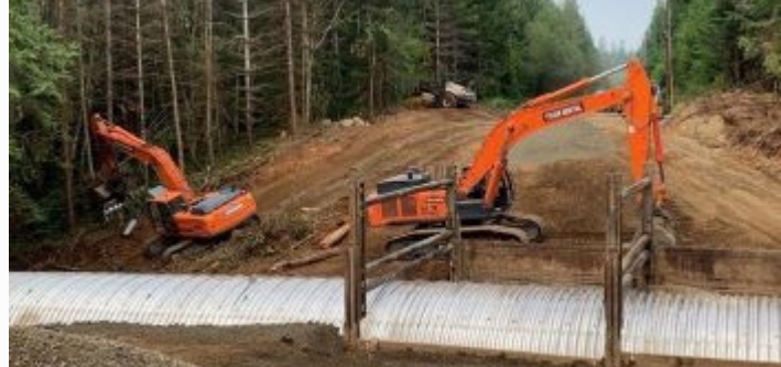
Above: Conway Construction in Shelton, WA working on a fish culvert replacement project.
