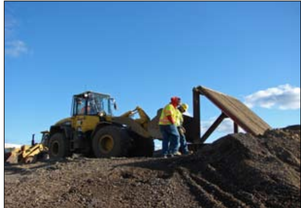
Planning the placement of the screen for the loader course
