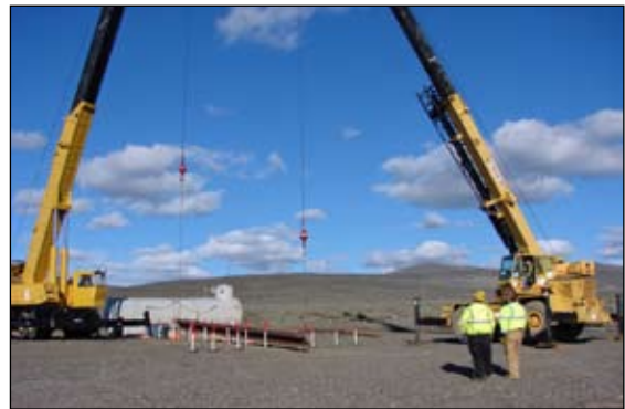
Practicing multiple crane lift planning and execution
