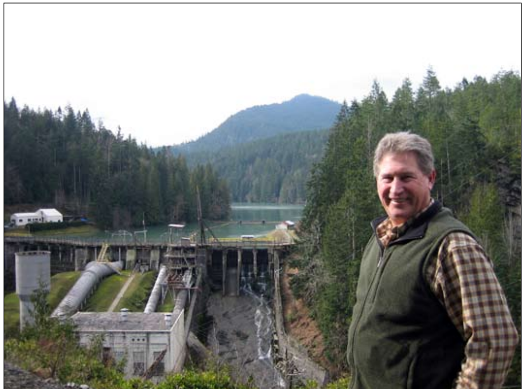
District 3 Representative George Garten and in front of the Elwha River Dam in the Olympic National Forest. The dam is slated for demolition in 2012. Bid proposal requests were sent out in mid-April, and the construction contract will be awarded by September 2010.
