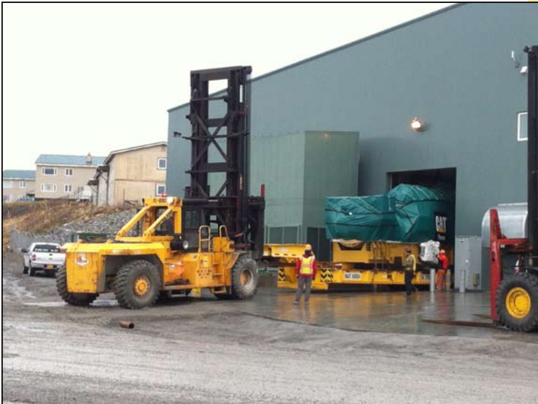
City of Unalaska Power Plant getting a new engine
