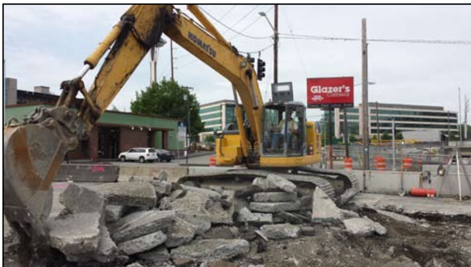
Ryan Harrison working for KLB on Mercer West project
