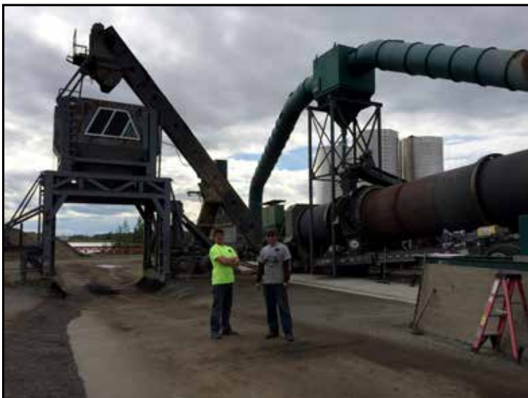
Mechanics Joe Beck and Kyle Krause at the Fairbanks Asphalt Plant - Paving Products Inc
