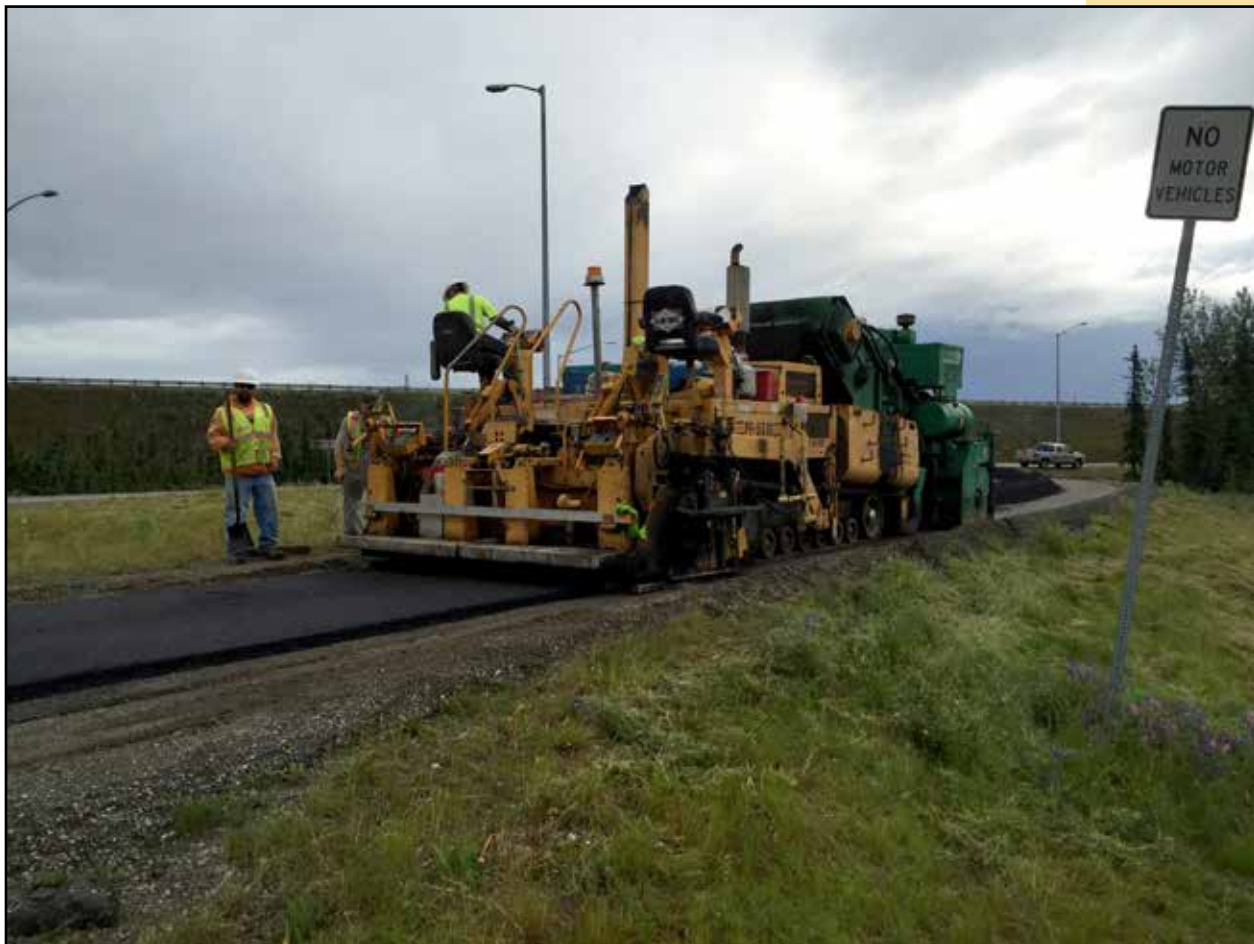
Exclusive Paving on Badger Road Bike Path
