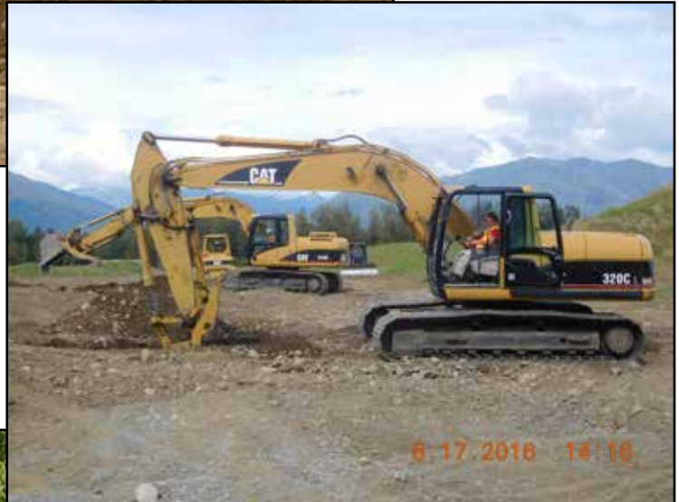
Women-in-the-Trades Excavator Training
