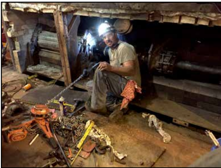
Doyon Utilities CHPP Boiler Front to Back Overhaul. Mechanic Cory Berg.
