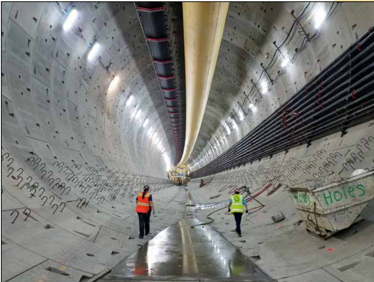
Lacey Hall and Marge Newgent approaching Bertha's trailing gear on the SR 99 tunnel project.
