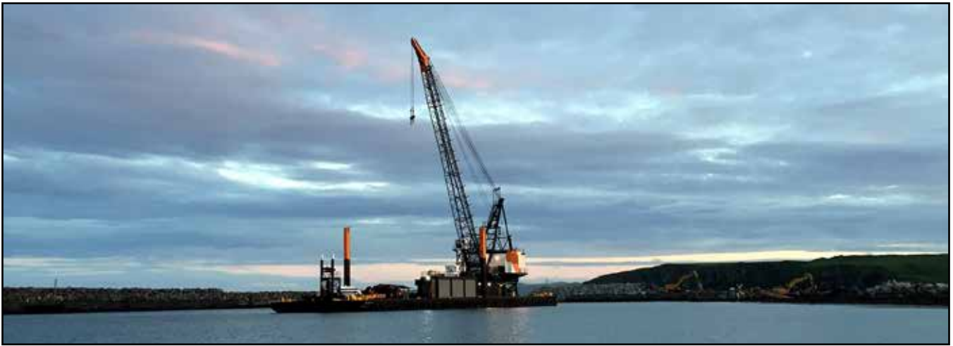
Crane Operators Kit Sundsten and Erik Sundsten in St. Paul Harbor.
