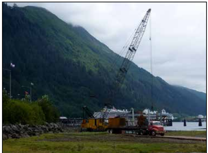
Jim Trucano – North Pacific Erectors – Juneau Sea Walk Project
