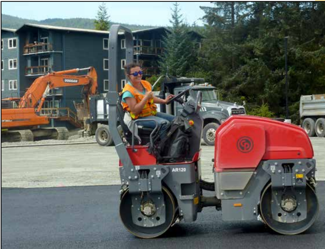
Nicole Carson Finish Roller for Miller Construction on Statter Harbor Project.
