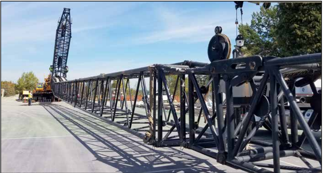
Ness & Campbell crew building the 550 luffing jib.
