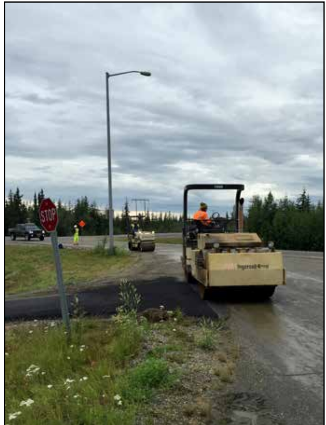
Exclusive Paving on Badger Road Bike Path
