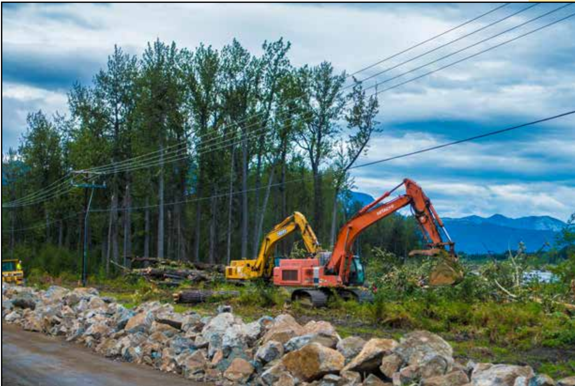
Granite Construction - Old Glenn Emergency Repairs
