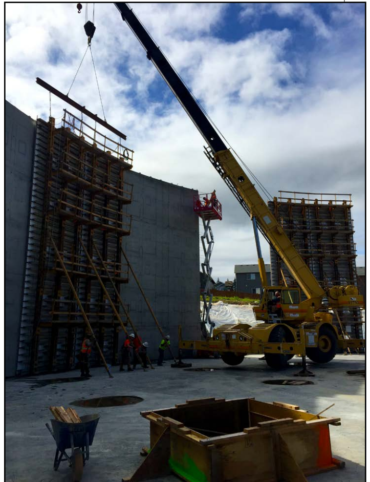
Brad Jevons working for Ward-Hindshaw Mt. Vernon Water Tower
