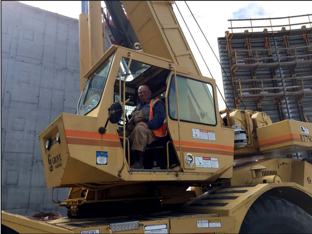
Brad Jevons at the Mt Vernon Water Tower working for Ward-Hinshaw
