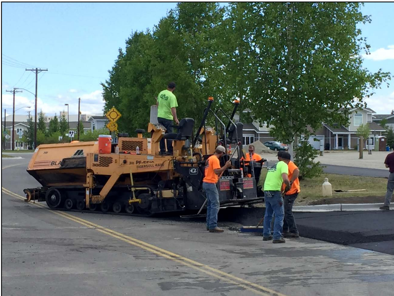
Paving Products - Fort Wainwright - Mike Carlson Topside - Tim Reese Screed
