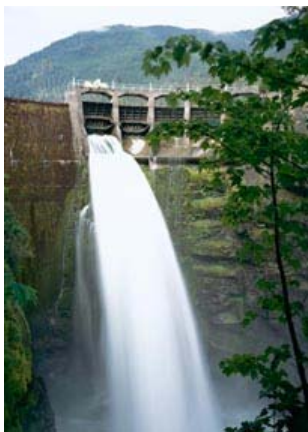
Glines Canyon Dam Photo by Scott Church
