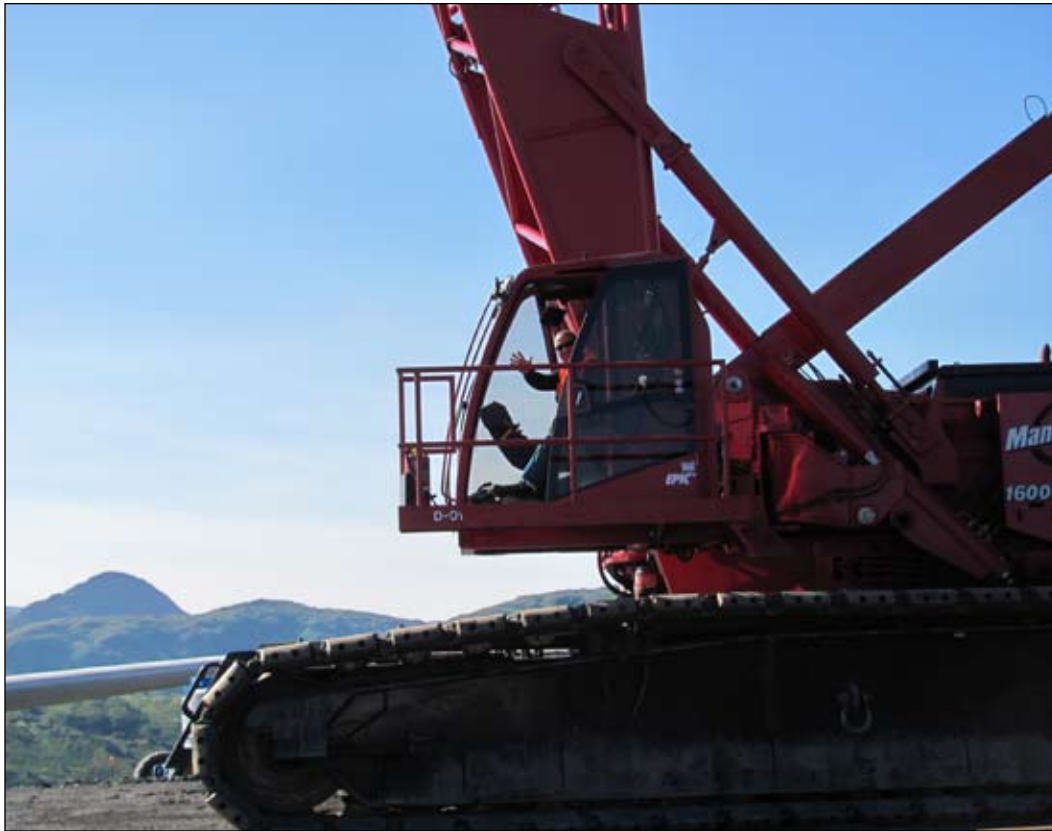
Kodiak Pillar Mountain Wind Turbine Project
