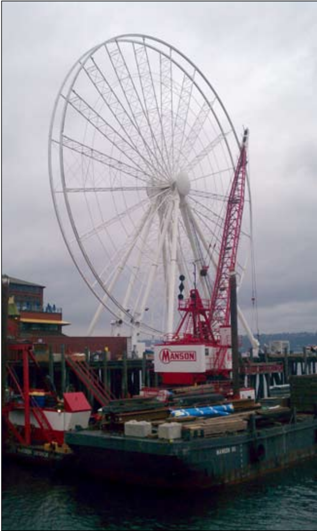
The Great Wheel - Manson Construction
