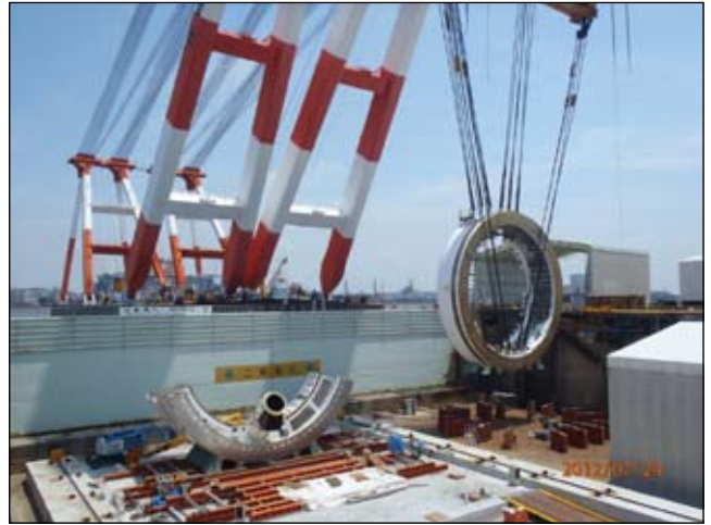
Worlds largest TBM being assembled for SR99 Deep Bore Tunnel
