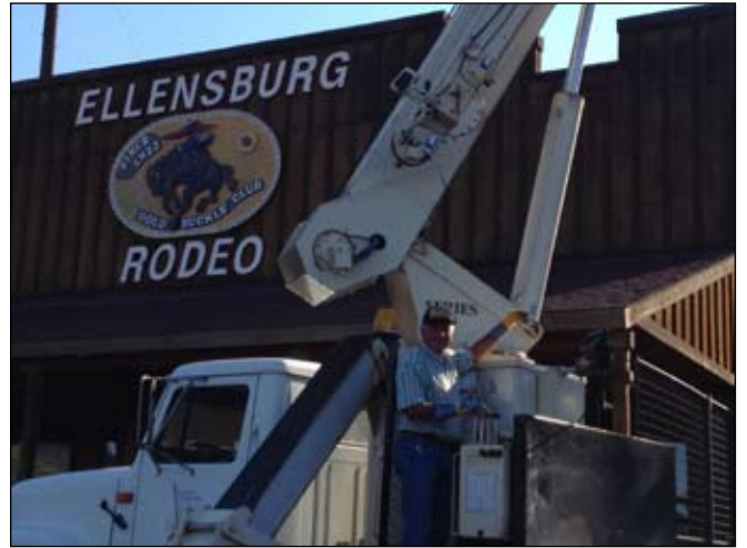
Above: Crane instructor Rick Wyllys, Operating a crane to set the scoreboard in the rodeo arena
