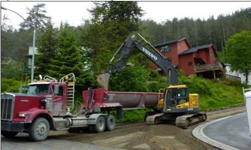
Operator Mike Corcoran loading trucks/ Channel Construction
