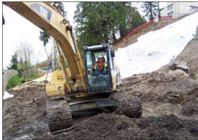
Rebecca Bechtold for Marshbank Construction on SR520 Easide Corridor.
