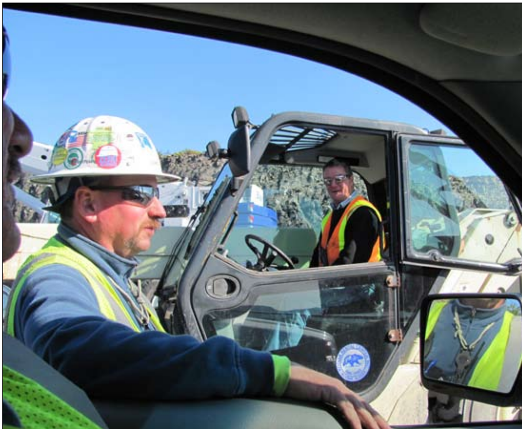
Kodiak Pillar Mountain Wind Turbine Project
