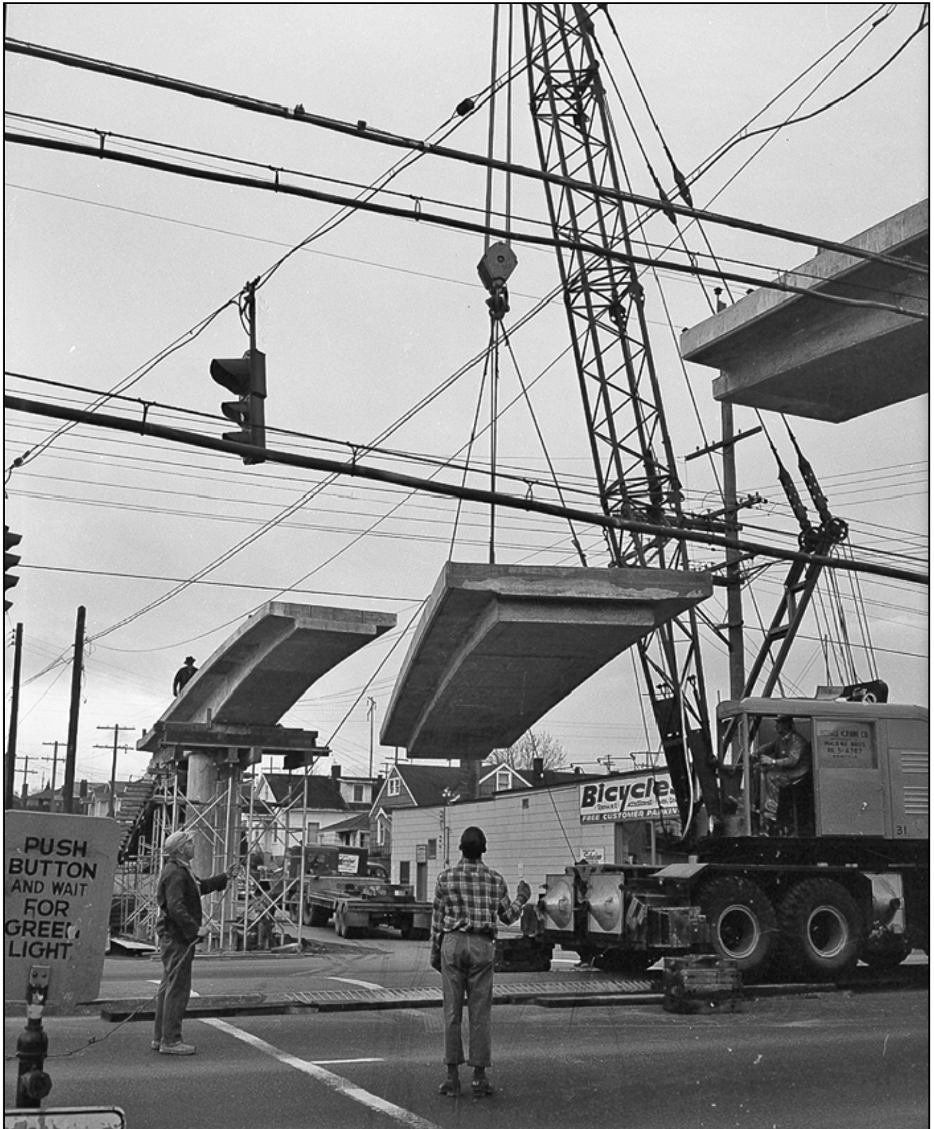
Construction of the bridge at Aurora and 102nd. 1961
