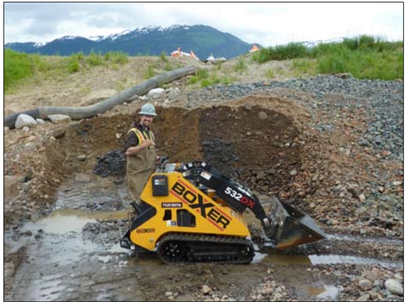
Operator Herman Collins/ Contractor AIC - Juneau
