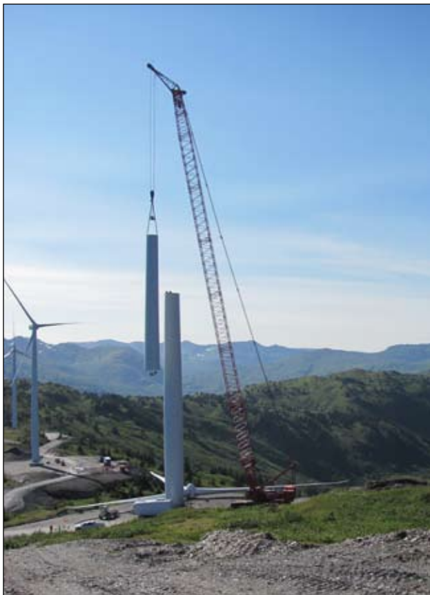
Kodiak Pillar Mountain Wind Turbine Project.
