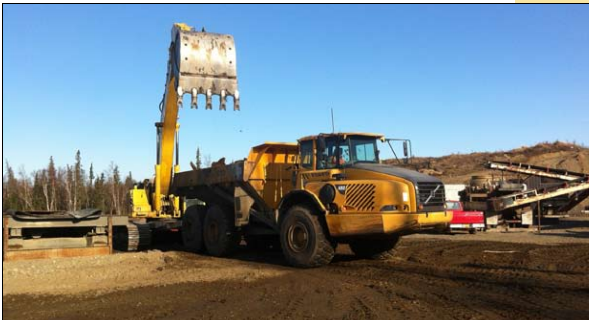
Loading off road haulers on Trunk Road phase 2, Wasilla Alaska
