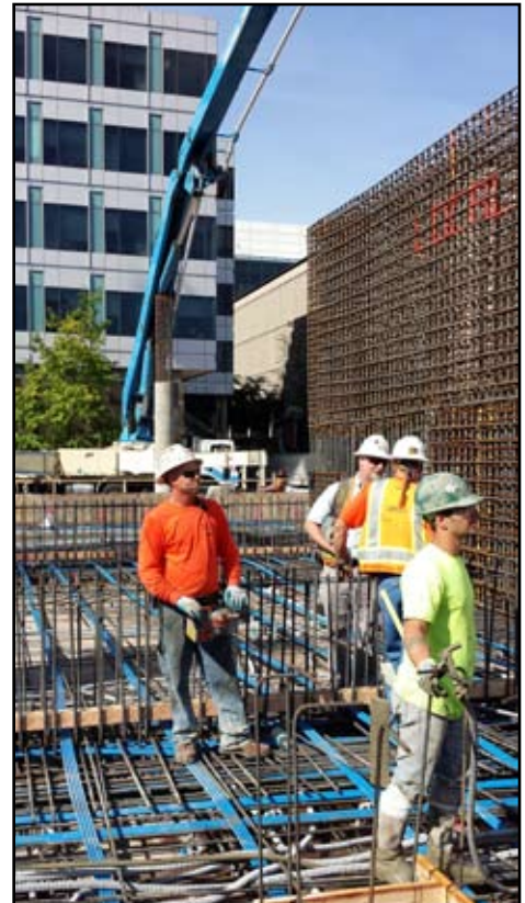
Jeremy Lytle - Ralph's Concrete Pumpers
