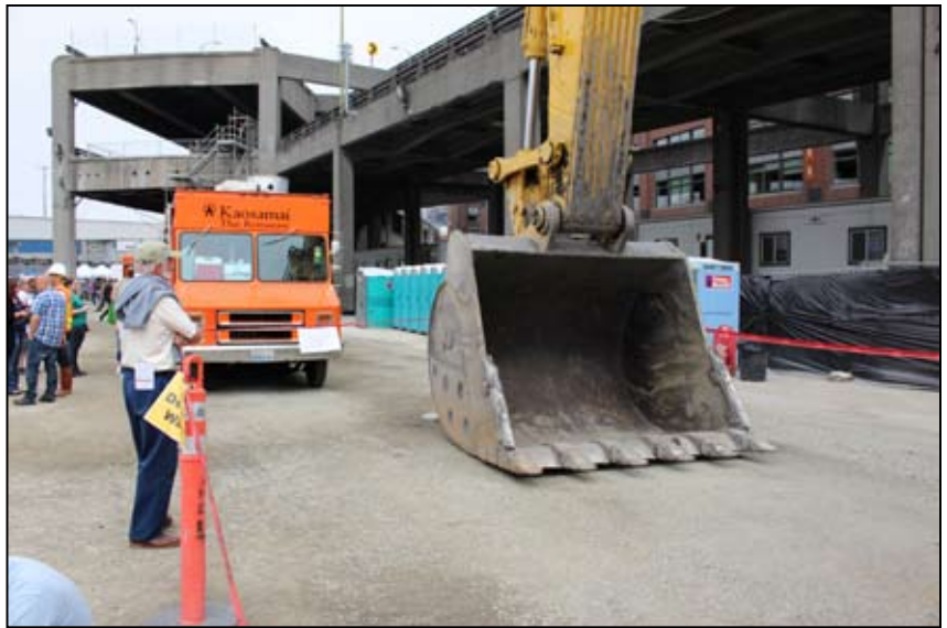
Press Day at the Seattle Tunnel Project
