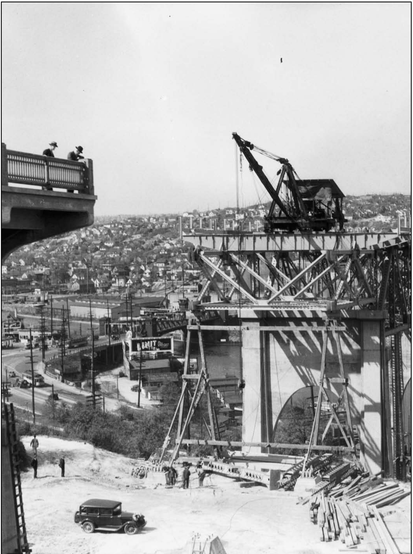
Aurora Bridge Construction 1931
