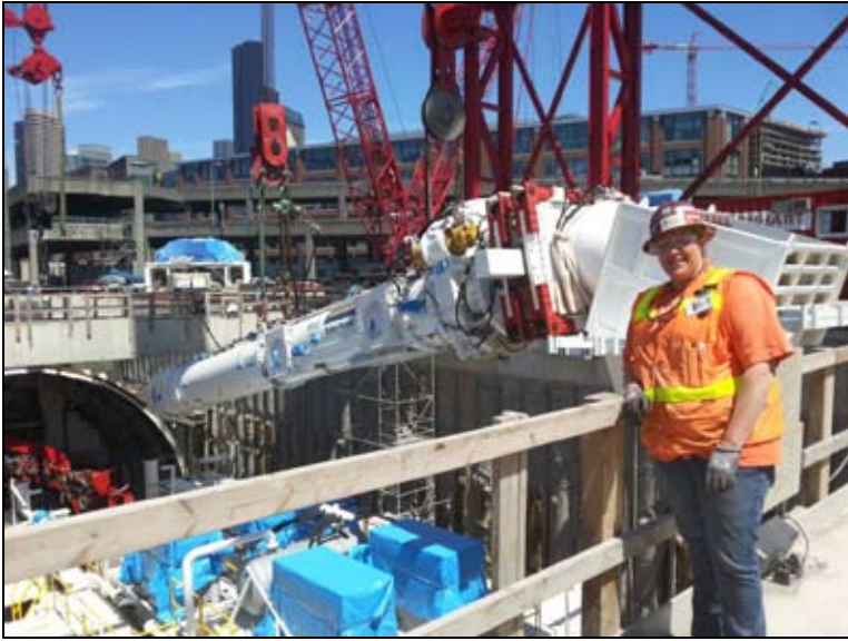
Jamie Willard - Seattle Tunnel Project
