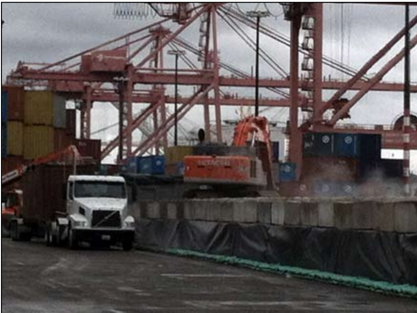
Dan Youso running the excavator on terminal 46 loading tunnel muck.
