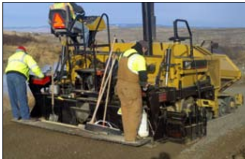
Learning to run screed in the Paving class.
