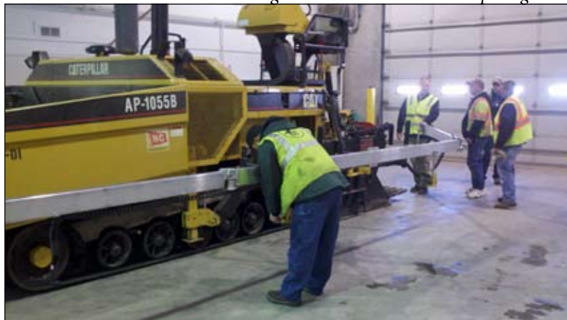
Checking out the automatics with the paving class.
