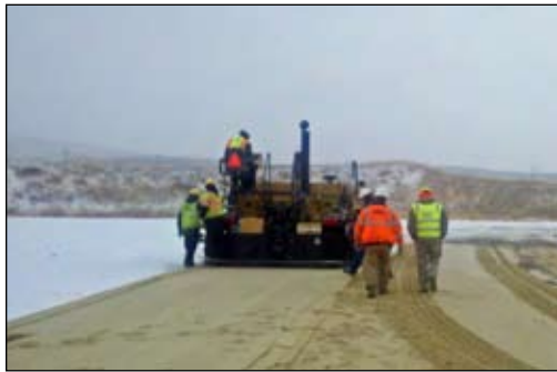
Paving over the winter weather.
