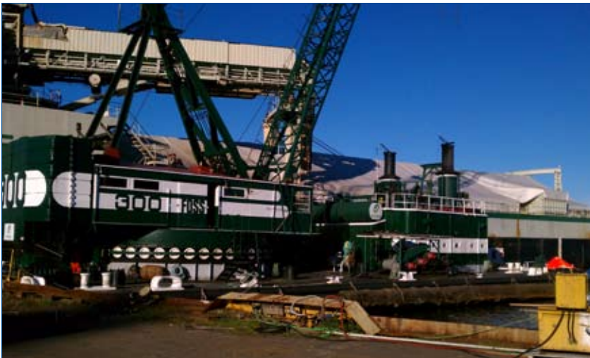
Pier 57 Manson Ferris Wheel Project
