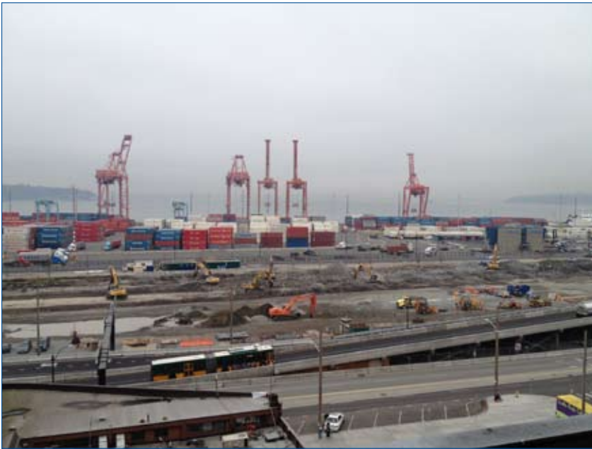
Viaduct Work in Seattle
