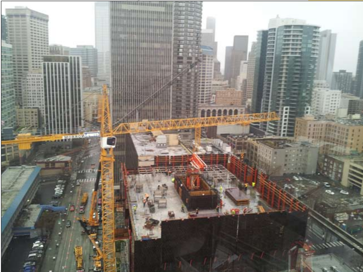
Lease Crutcher Lewis - Twin 20 Story Apartment Towers in Downtown Seattle
