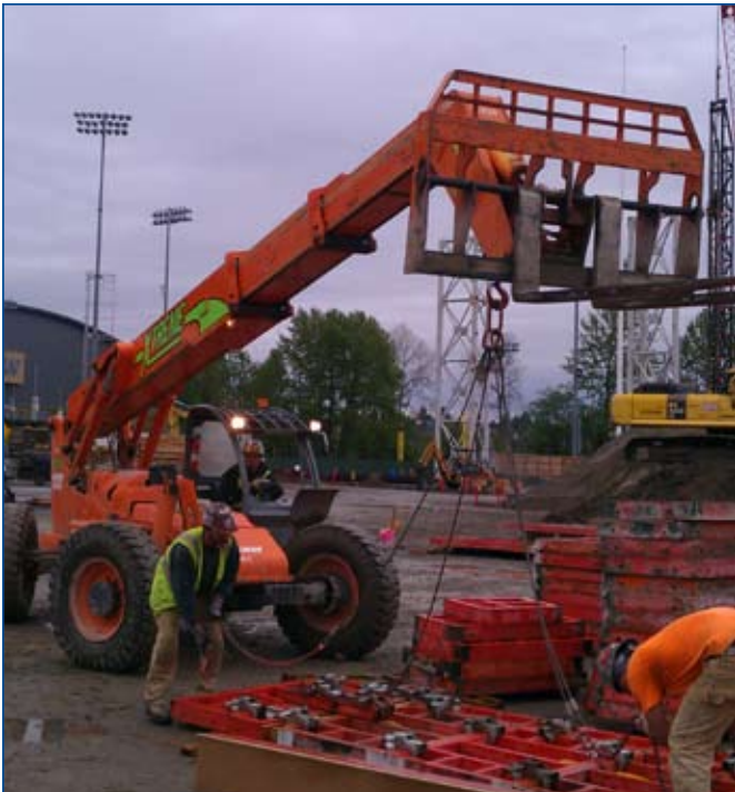
Husky Stadium - Joel Kienitz Turner Forklift
