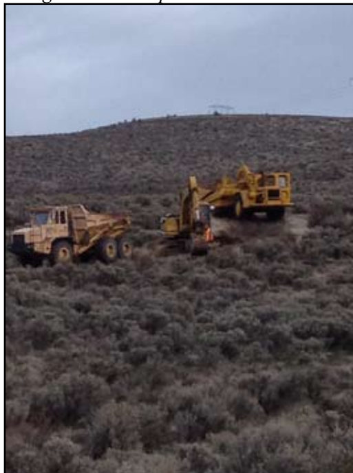
Using the new scraper
