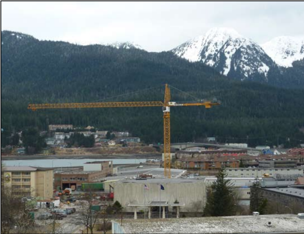
Tower Crane in Juneau Alaska
