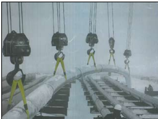
Replacing pipe in Prudhoe Bay, Alaska From Archives
