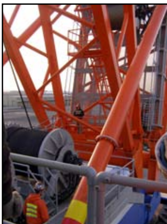
The view from on the crane itself
