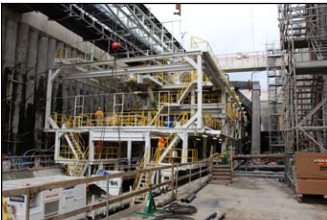
SR99 TUNNEL PROJECT
