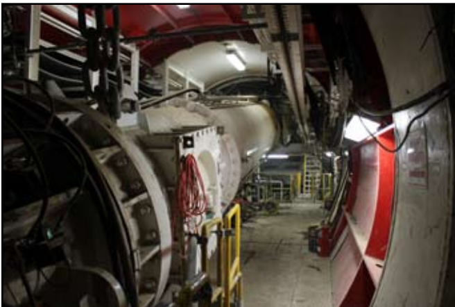
SR99 TUNNEL PROJECT
