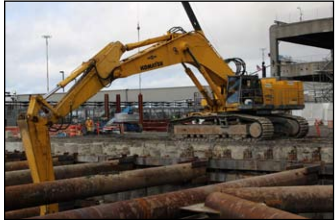
Kyle Kayser - SR99 TUNNEL PROJECT
