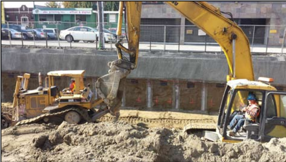
Hoss Bros. 1st & Thomas St. Mass excavation
