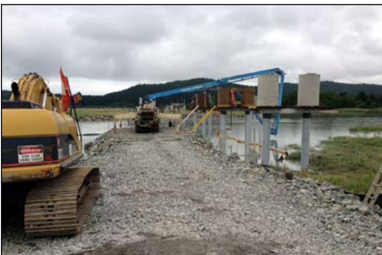
Pumping the north end landing lights for the Juneau airport
