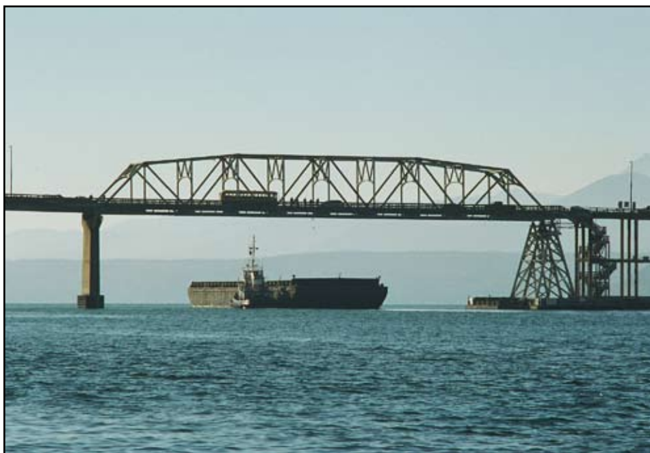
A typical barge transiting the eastern span of the Hood Canal Bridge as proposed.
