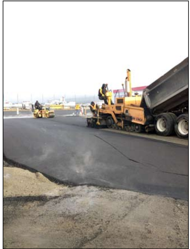
Paving project at the Fairbanks Airport
