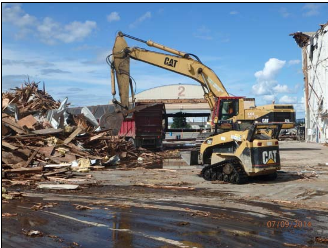
Central Environmental - Taking down hangers built during WWII on Ft. Wainwright.
