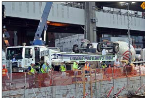
Waterfront Seawall Construction
