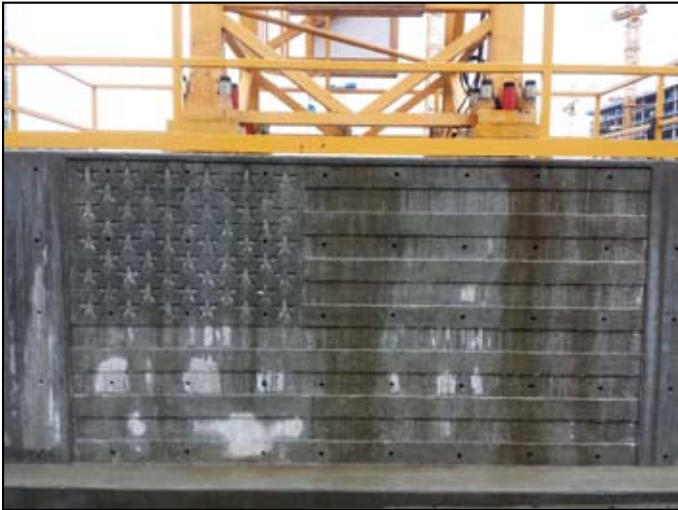
Lease Crutcher Lewis American Made Tower Crane Base
