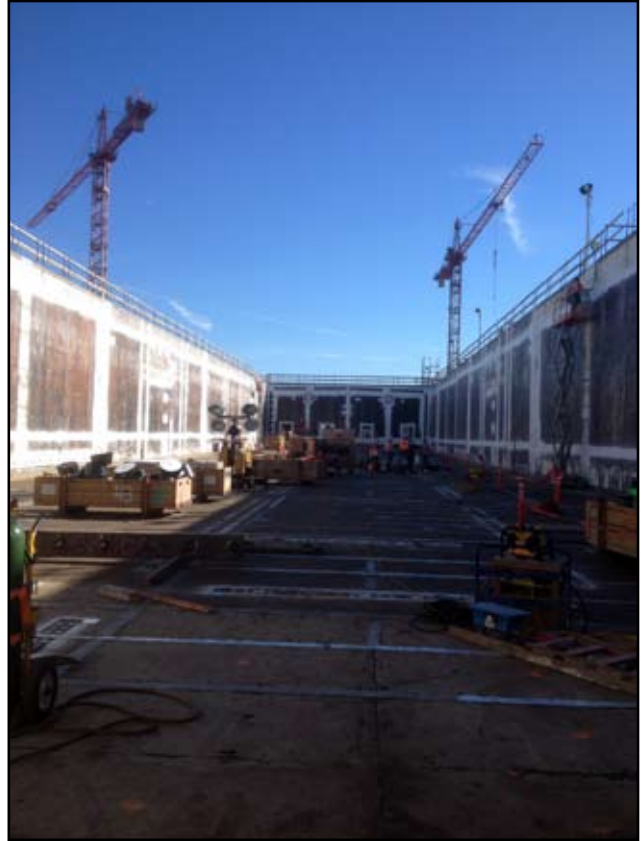
Casting basin for SR-520 pontoons in Aberdeen
