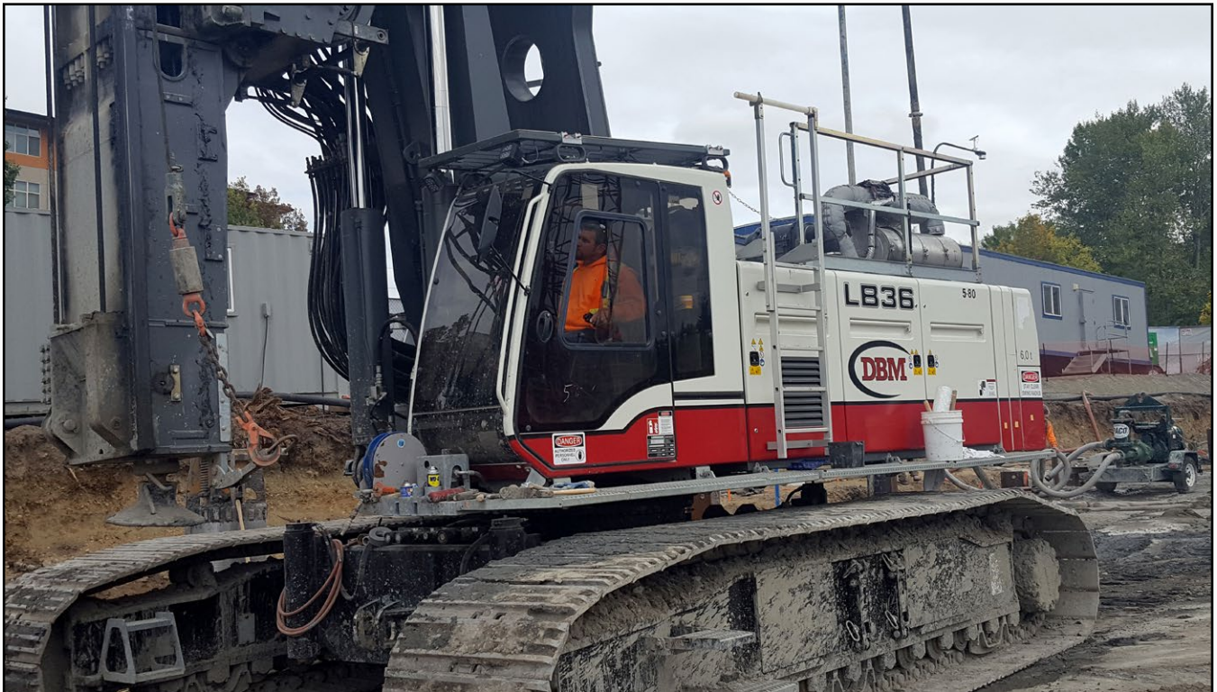
Tom Gallichan drill operator for DBM
