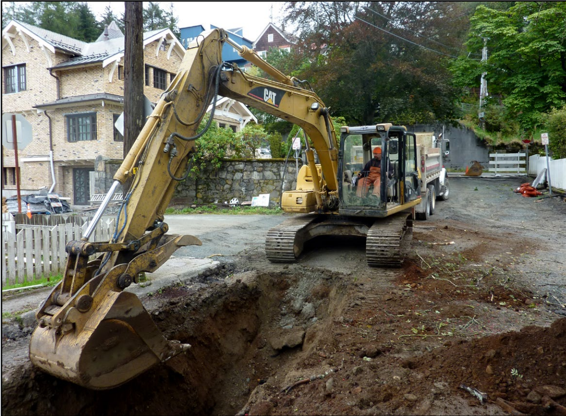
Shaun Lewis working for Admiralty Construction
