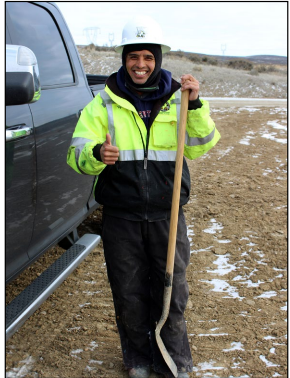
Dozer instructor Efrain Saucedo with his great, "can do" attitude and the track shovel going to show the apprentices how it's done.
