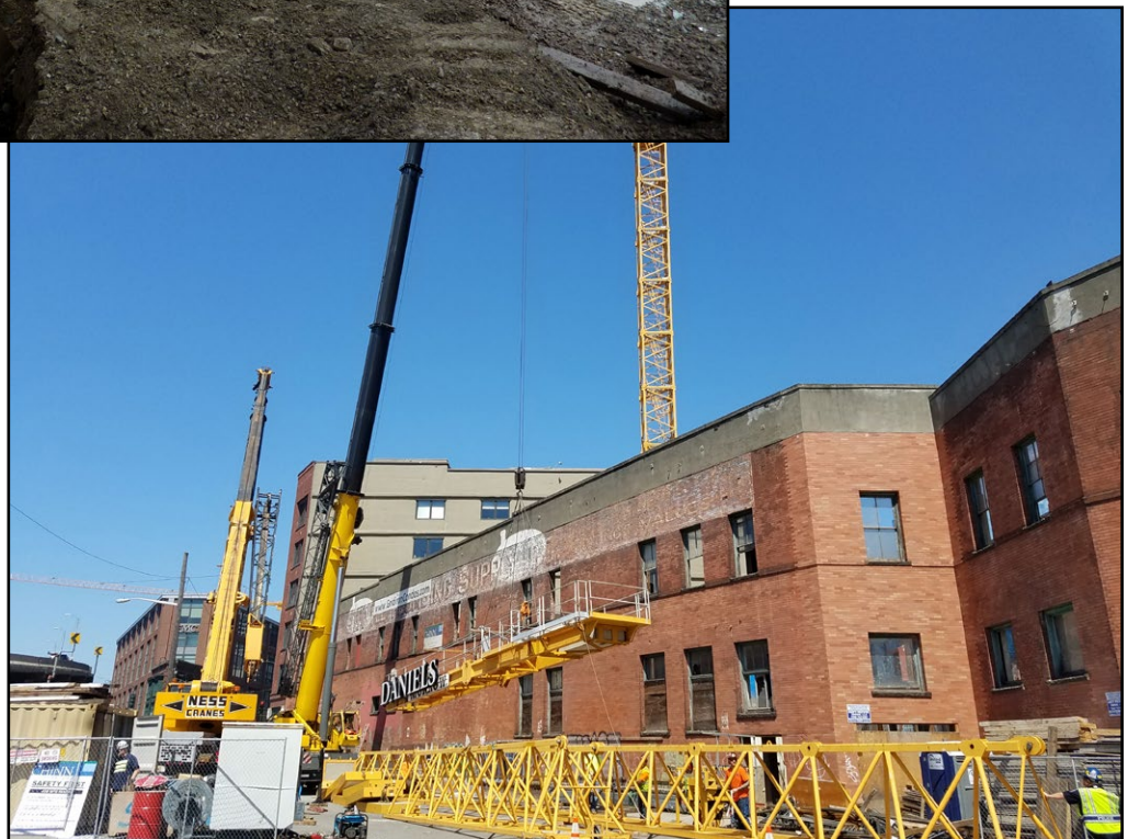
Ness & Campbell crane building another tower crane for Garner Construction
