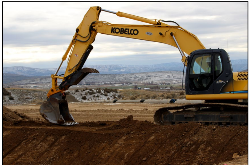
Apprentice Ben Burke carefully cleaning up the edge of his slope during this day's digging task in the excavator class
