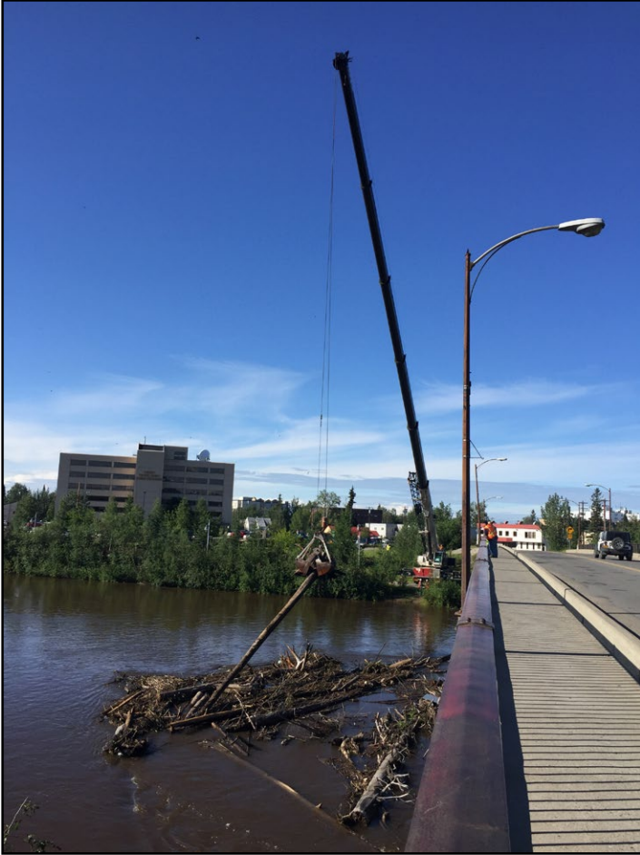
Precision Cranes removing debris and drift from the Chena river at the Wendall Street Bridge
