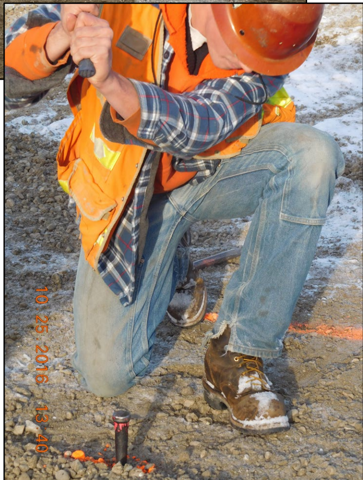
Apprentice, Destry Lietz preps to set a hub in grade-checking
