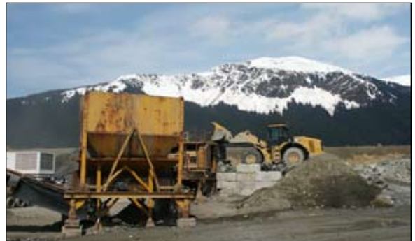
Plant operations in Alaska
