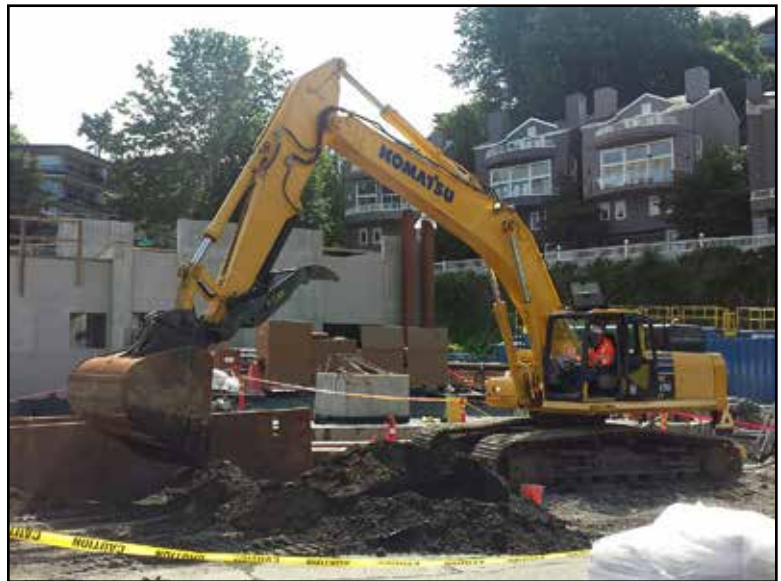
Paul Olson running the excavator at the Murray Pump Station
