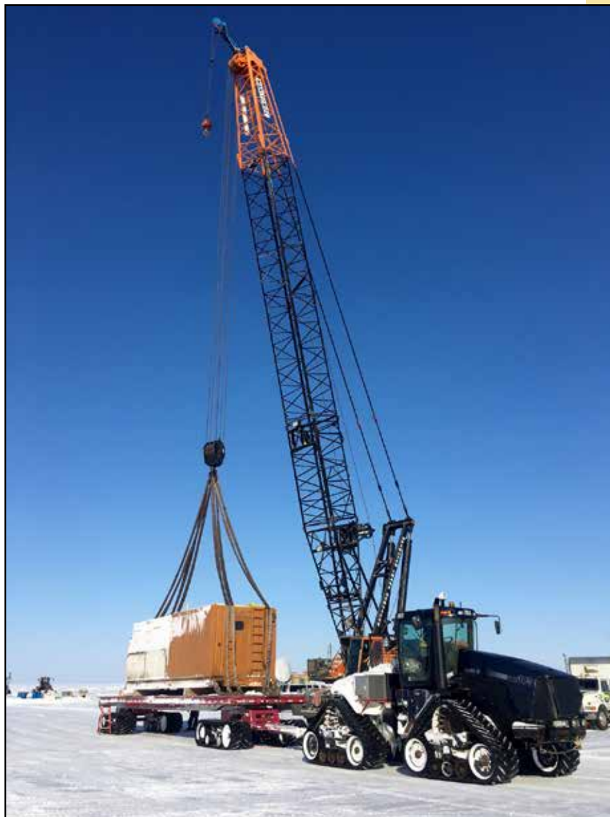
Cruz Construction and Northstar Equipment Services Submitted by Keegan Busse
