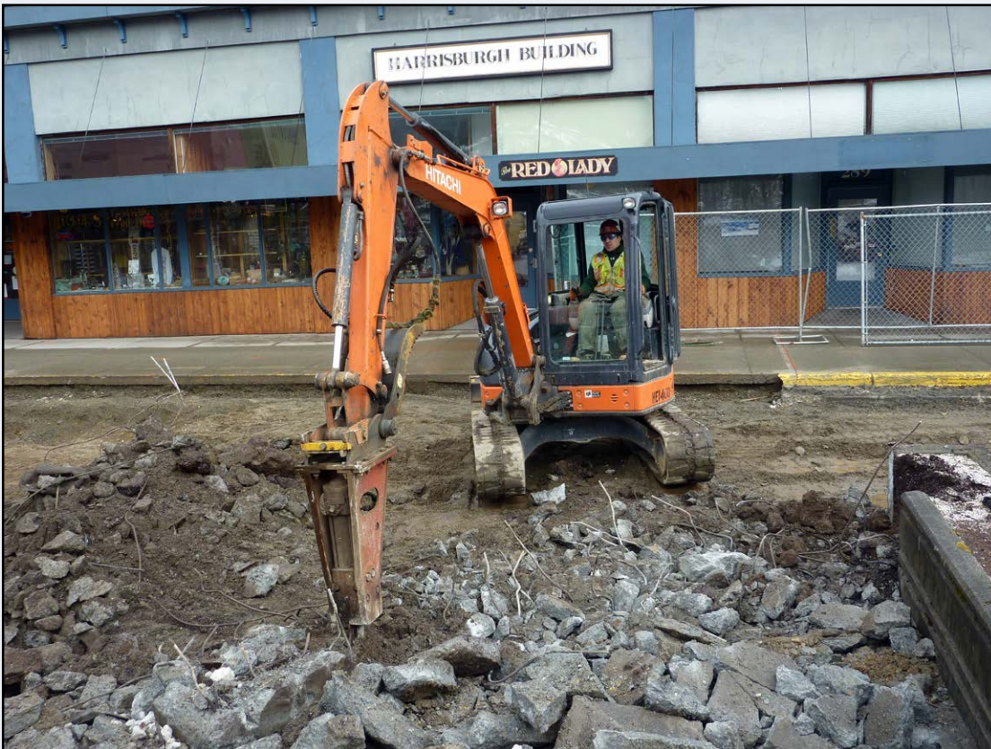
Apprentice Kory Hasbrouck working for Arete Construction
