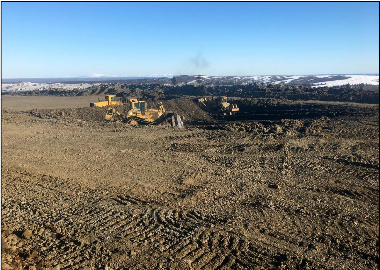
Phil Bungart and George Tugatuk ripping and stockpiling, with Rex Nick in Loader at the runway material site
