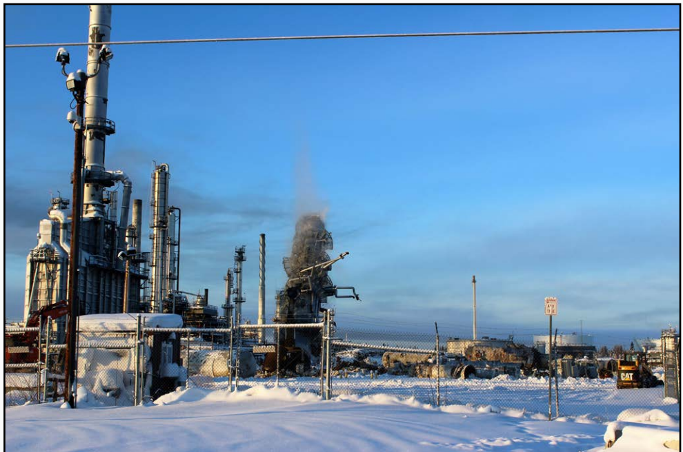
Demo on the North Pole Refinery project
