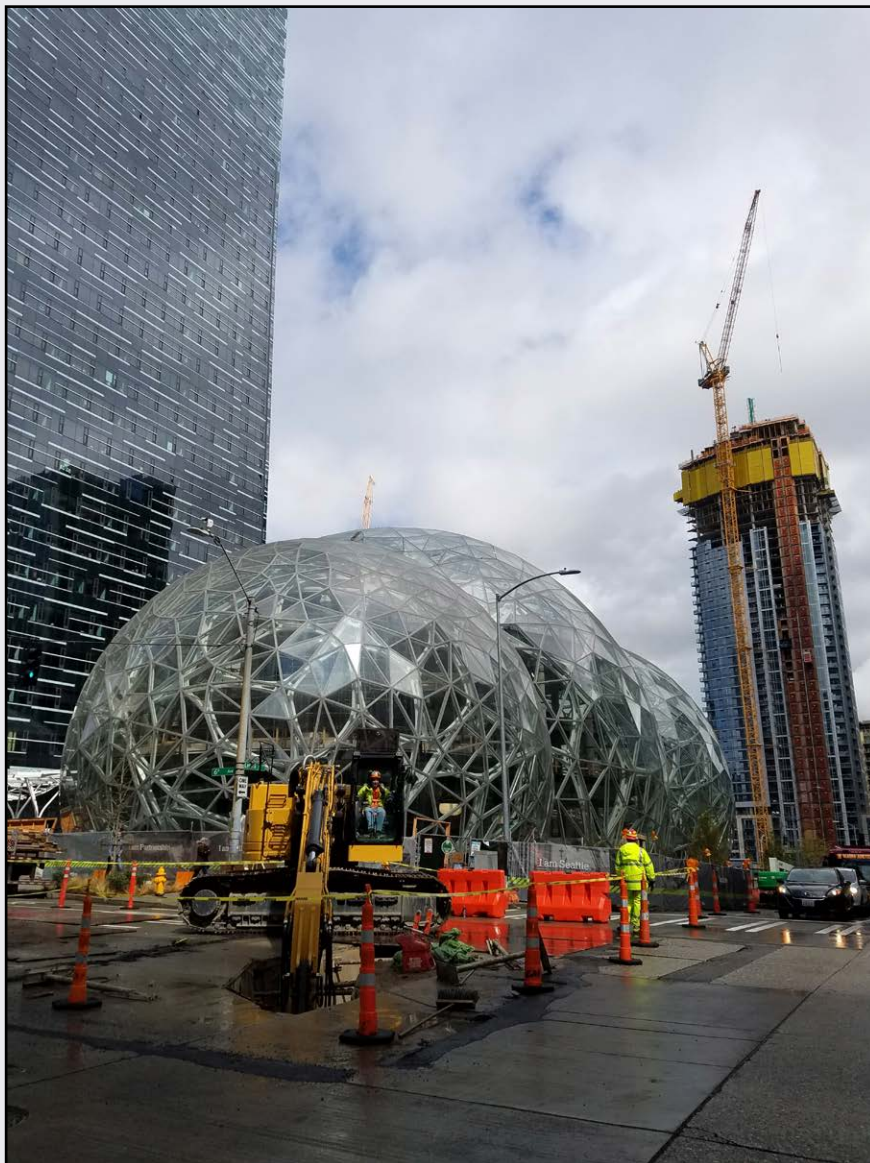
Galen Kindle running the excavator for Merlino – 6 th and Lenora
