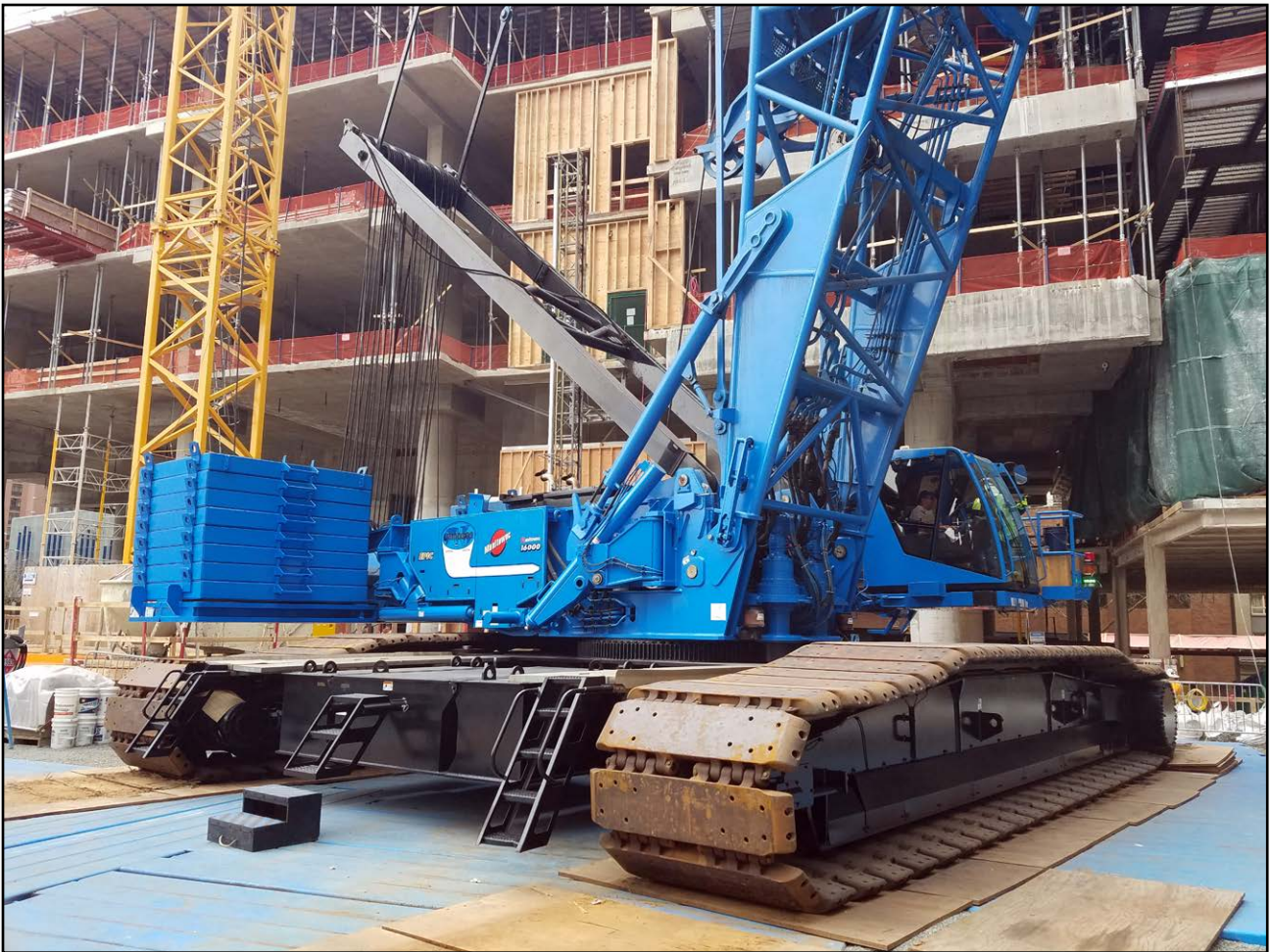
Dan Youso on the 16,000 for the Erection Company and Sellen
