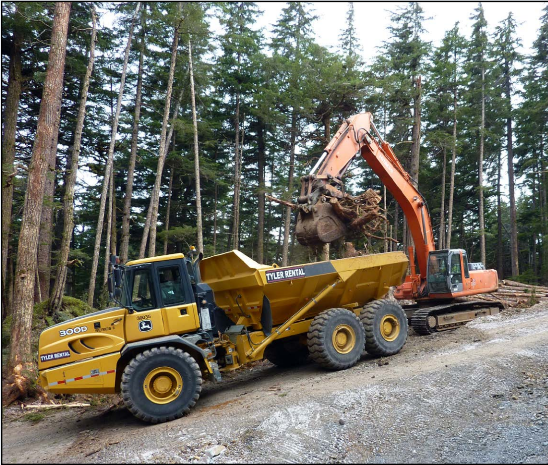
Rodger Engen working for Enco Construction
