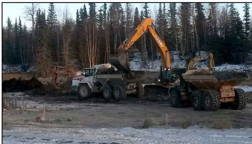
Students operate A.D.T's and excavators during January skills upgrade course
