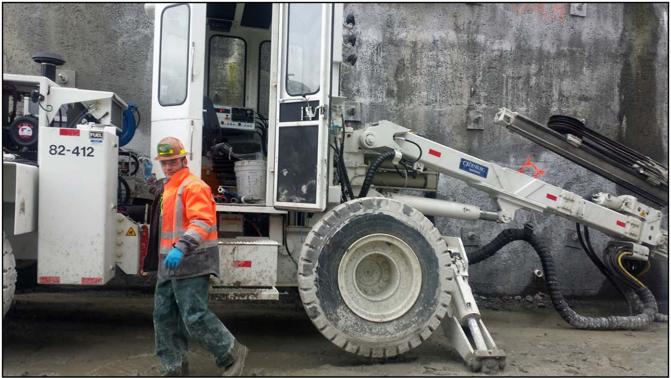
Joe Valleroy runs this Jumbo for Atkinson on the Bellevue Tunnel
