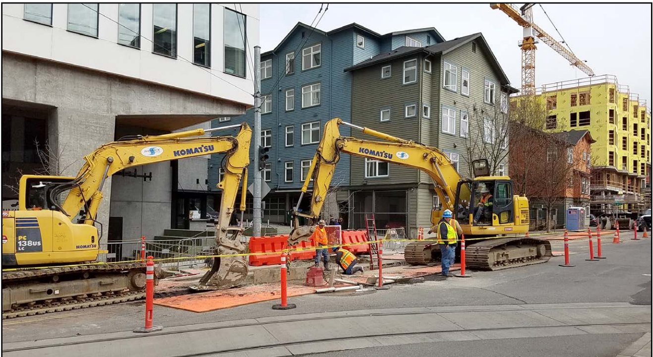
Schimik Construction - Denny Network - Power Upgrade on about 40 Blocks
