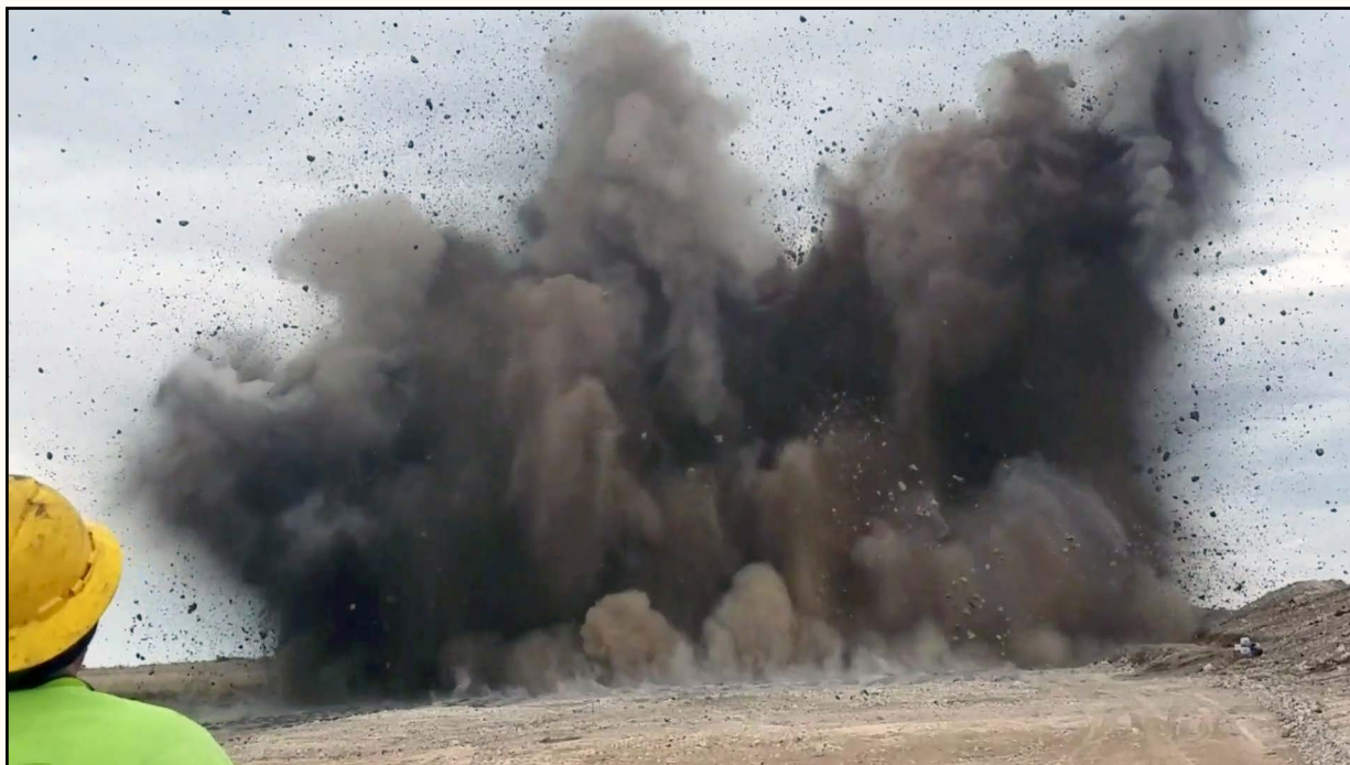
Western Construction Blasting at the pit in Spencer, Idaho
