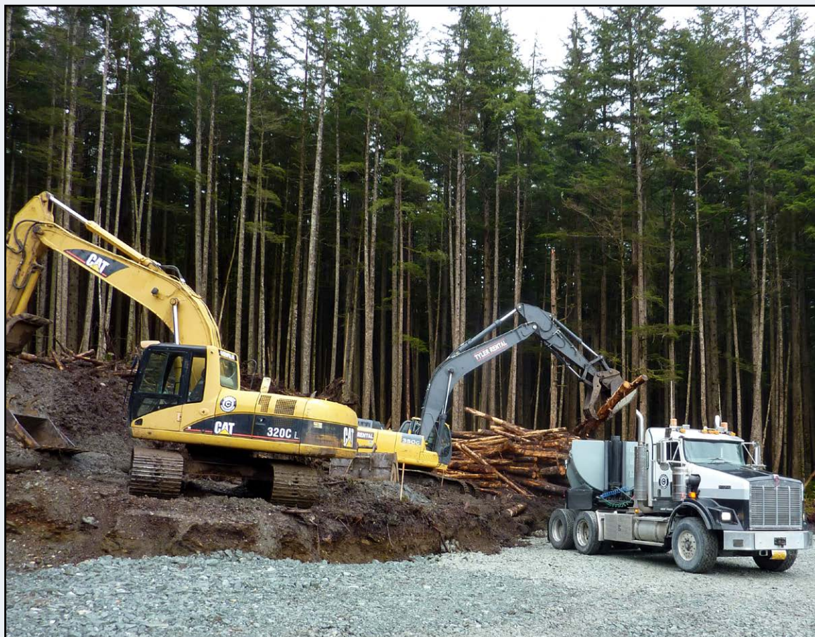
Jaret Reid loading logs into trucks for Coogan Construction
