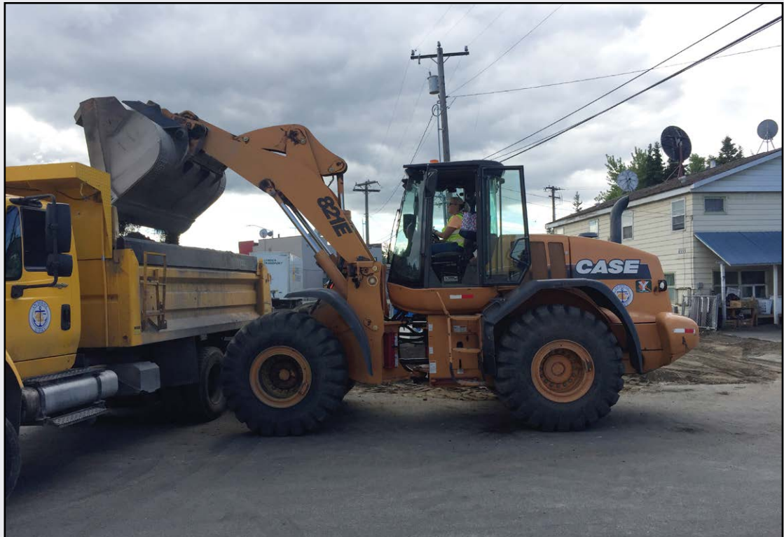
Michelle Stone - Prepping an alley for new asphalt - Municipality of Anchorage
