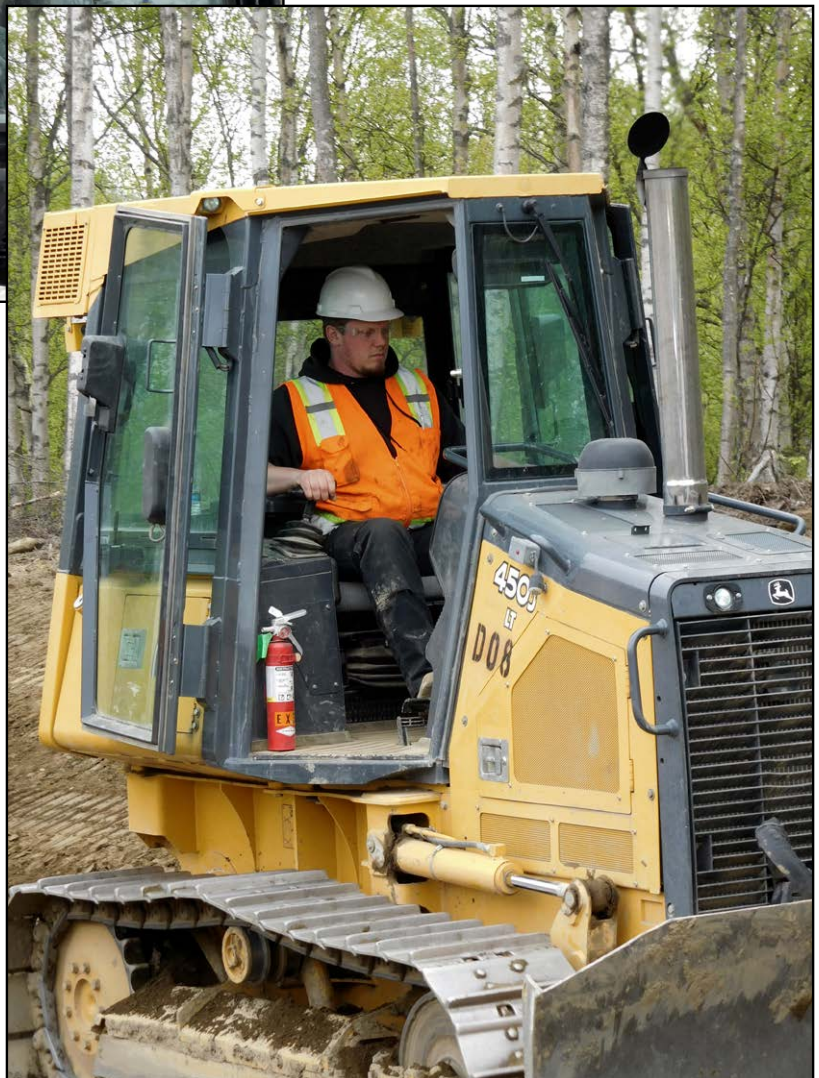
First year apprentice Bryan Dalbeck fine grading top-soil in the J.D. 450
