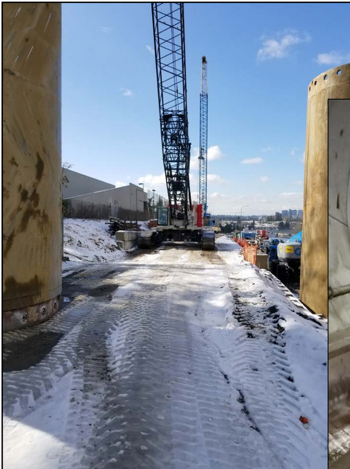
Malcolm Drilling - E 360 Kiewit/Hoffman project off 520 and 148th st
