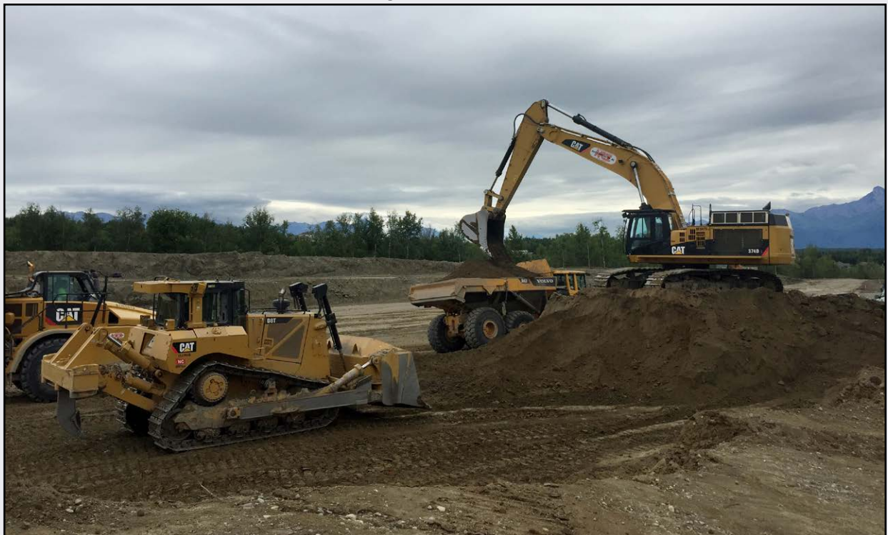
David Young, Neeser Construction Trunk Road Extension – Wasilla AK
