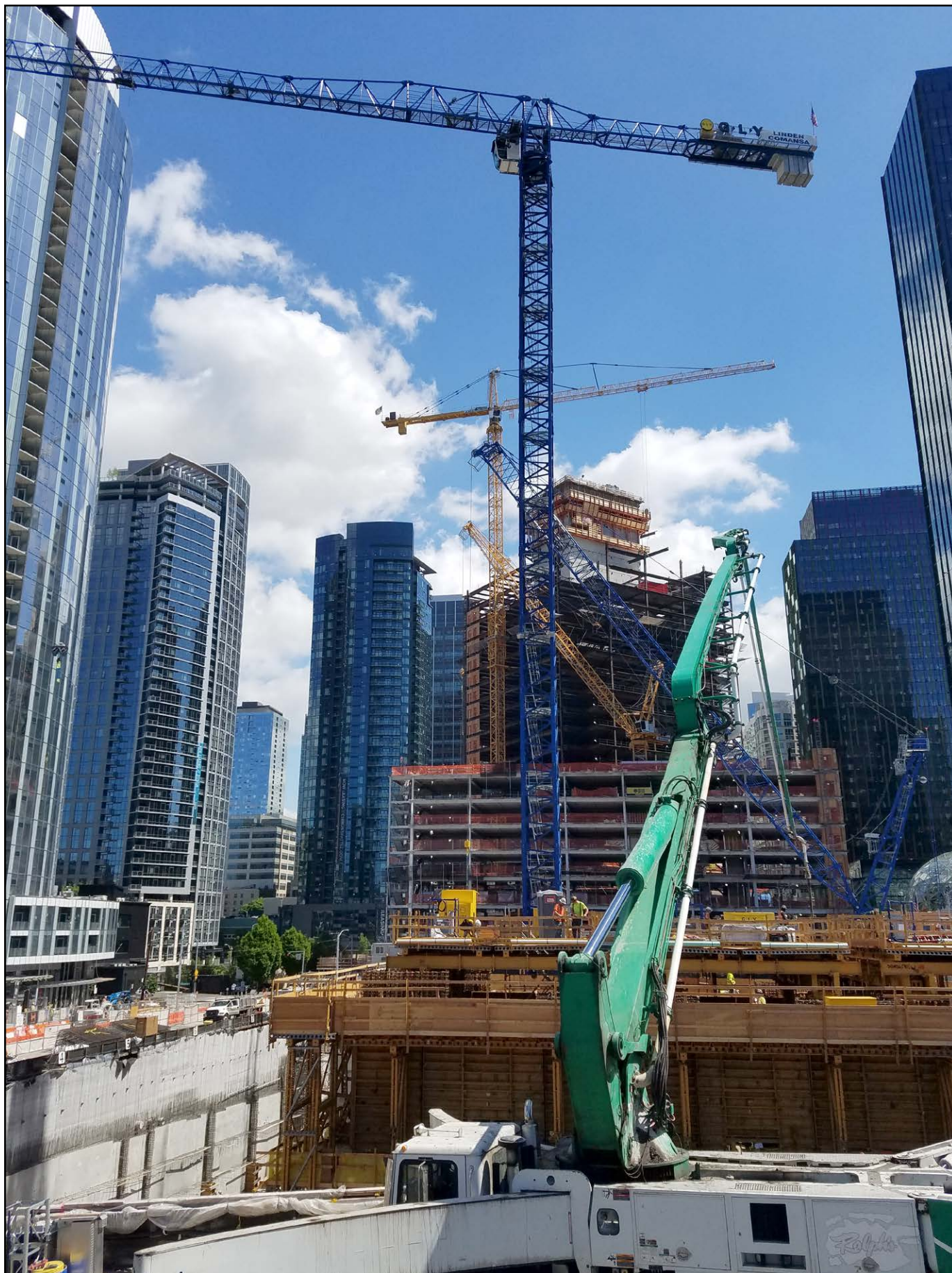
Several Operating Engineers working on the Amazon neighborhood in Seattle.
