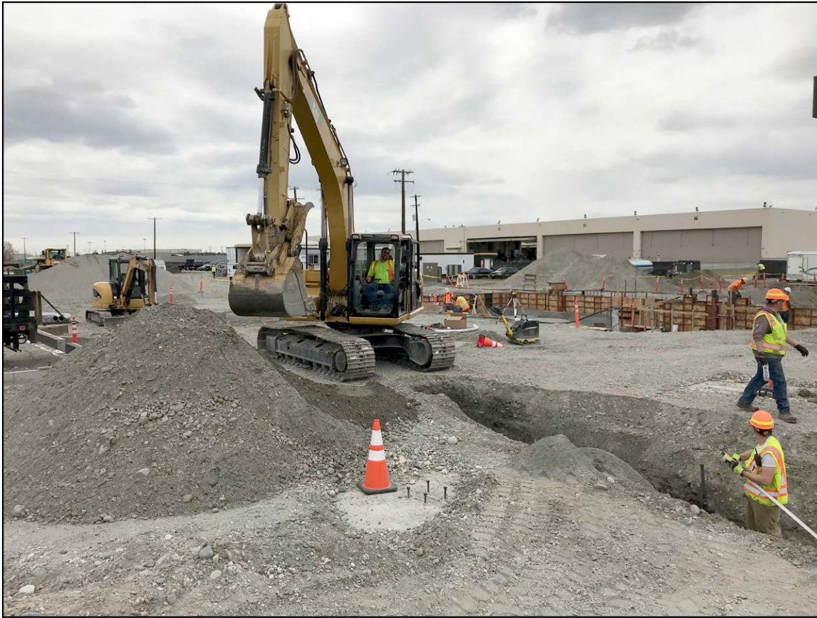
Prosser & Dagg - Ty Auvil on Excavator
