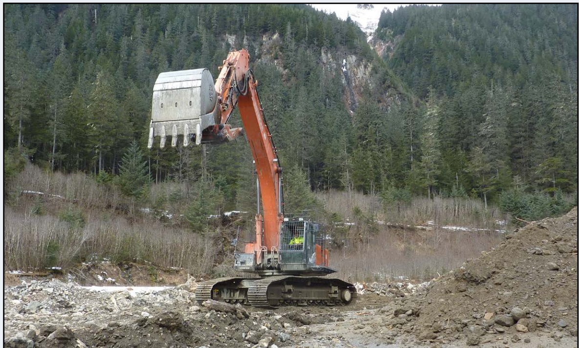
Todd Tucker with Secon Construction
