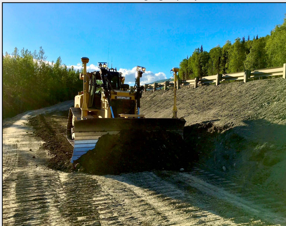
Sterling Highway Project - Granite Construction
