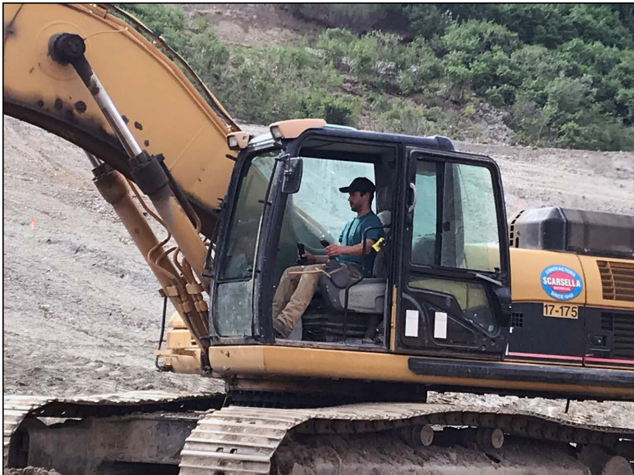
Apprentice Doran Sanford loading trucks - Scarcella Brothers - Healy reclamation project
