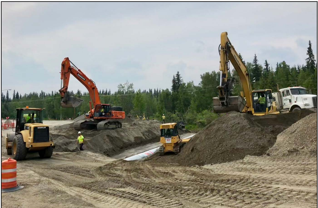
Exclusive Paving project on Farmers Loop Rd in Fairbanks, AK
