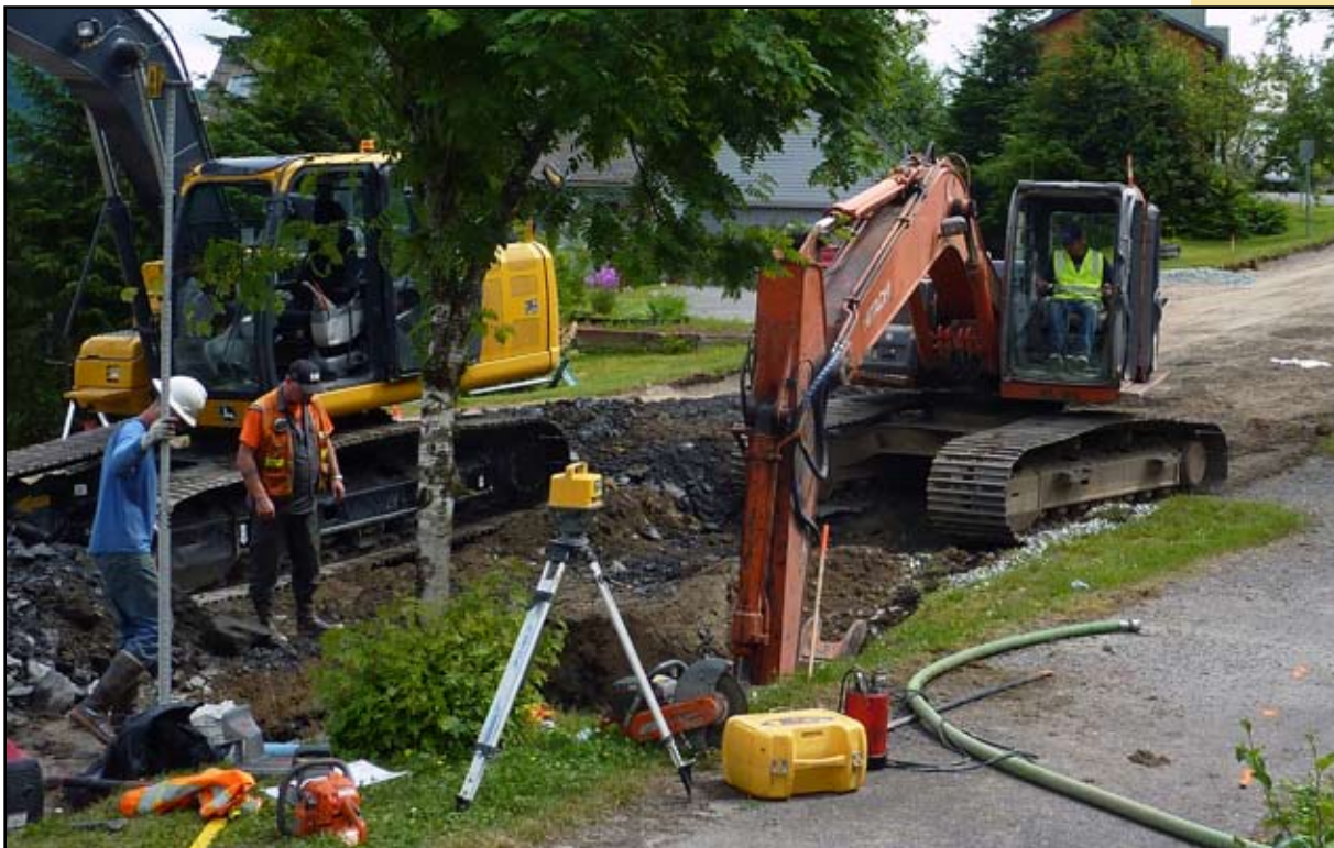
Todd Tuckers and Izzy Compos working for ENCO Construction.
