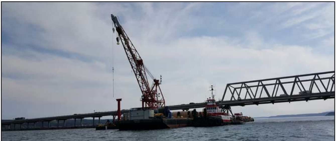
Manson working on the anchor cables on the Hood Canal Bridge
