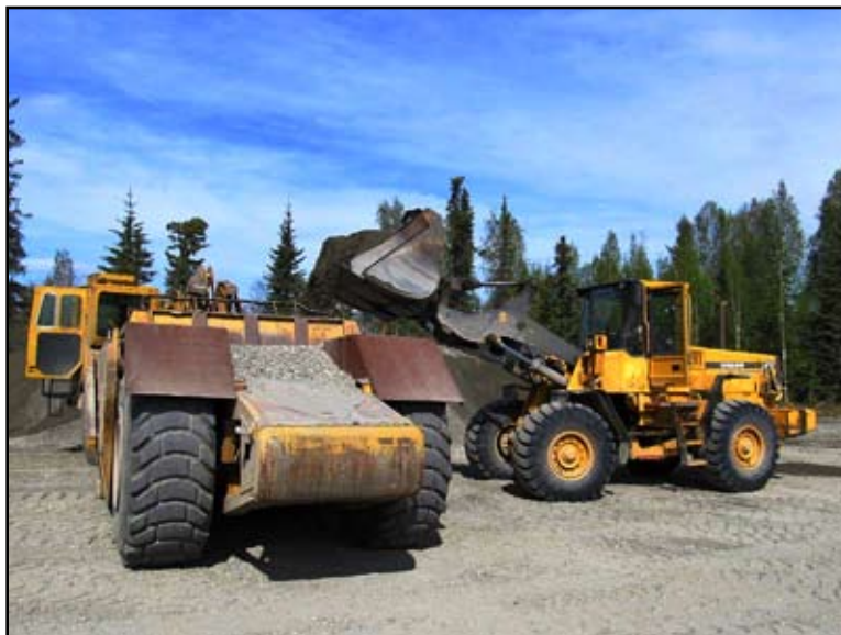
The old scraper and new front-end loader
