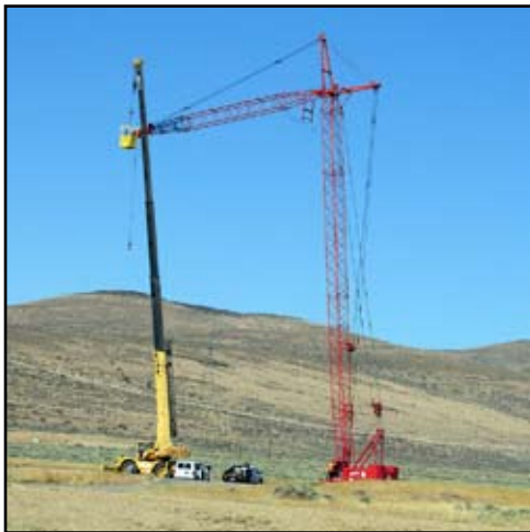
Putting together the luffing jib for the 222
