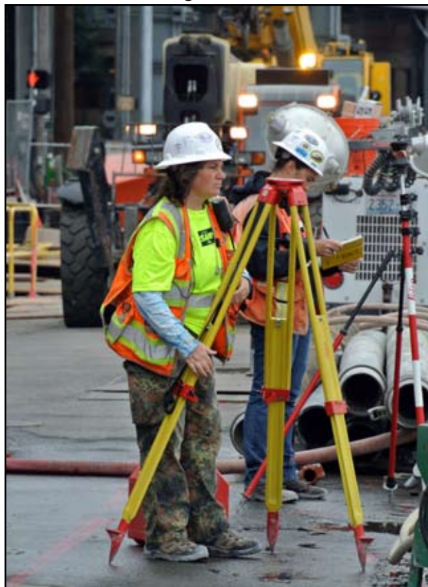
Dana Miller working on the Seawall for 1 Alliance
