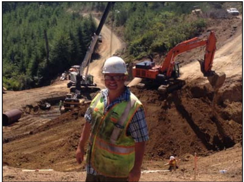
Benji Howard working on the Rock Crusher Hill Project
