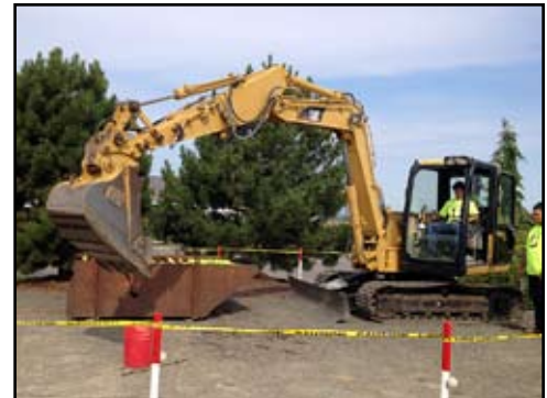
The Excavator for friends and family to try out
