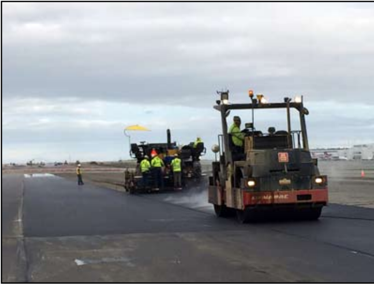
Granite Construction paving at the Anchorage International Airport
