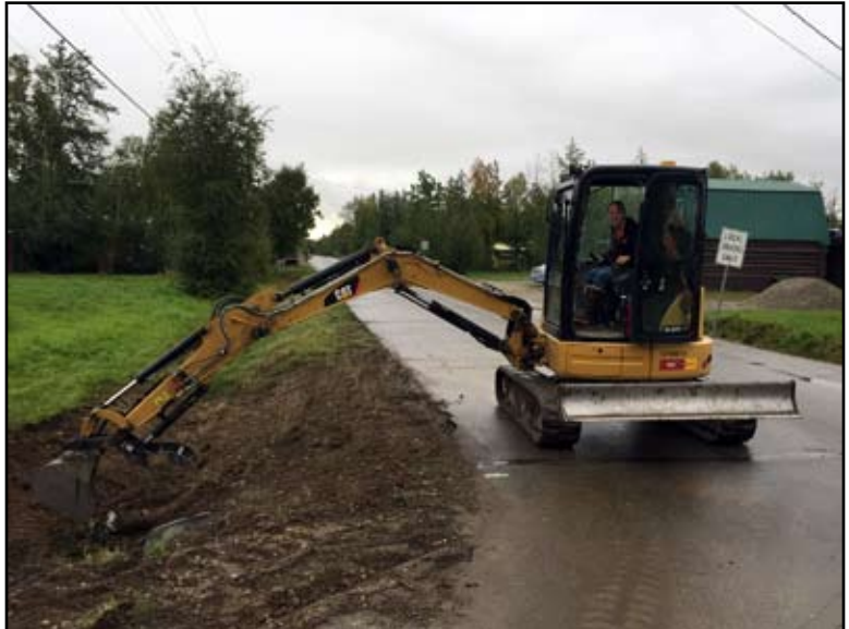
Melissa Albright finishing slopes for CEI, LNG distribution project North Pole
