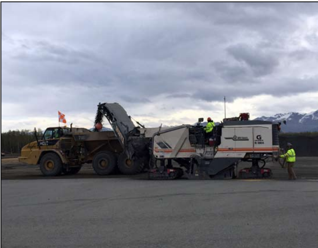
Granite Construction's Anchorage International Airport Job
