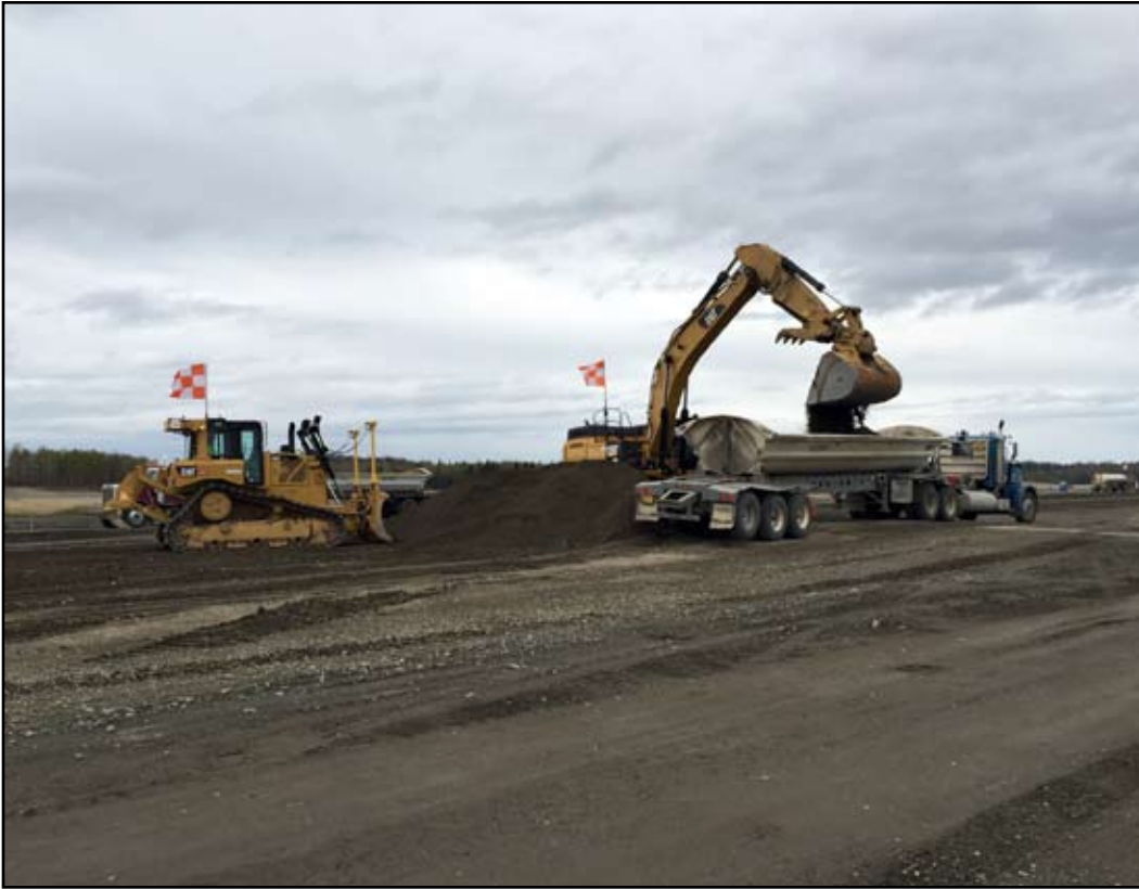
Granite Construction - Anchorage International Airport
