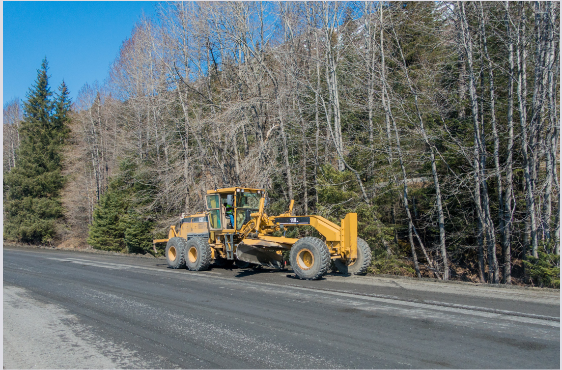
Owen Van Orman, Granite Construction, on the Seward Highway
