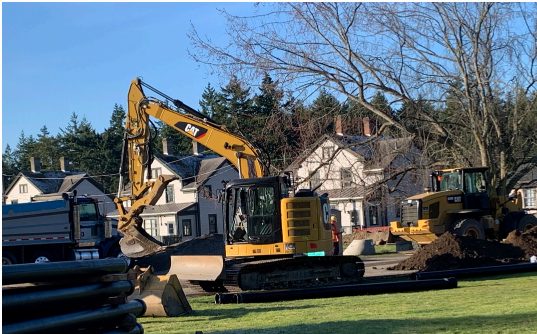
ICI at Fort Worden State Park. Wally Huntingford on excavator
