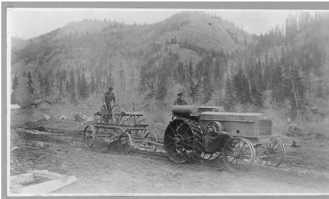
Grading in Tanana Valley around 1910
