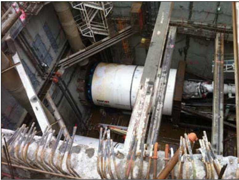
TBM at Sound Transit
