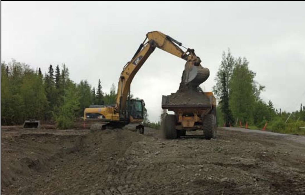
Scarsella Brothers – Machen Road Extension, Wasilla AK
