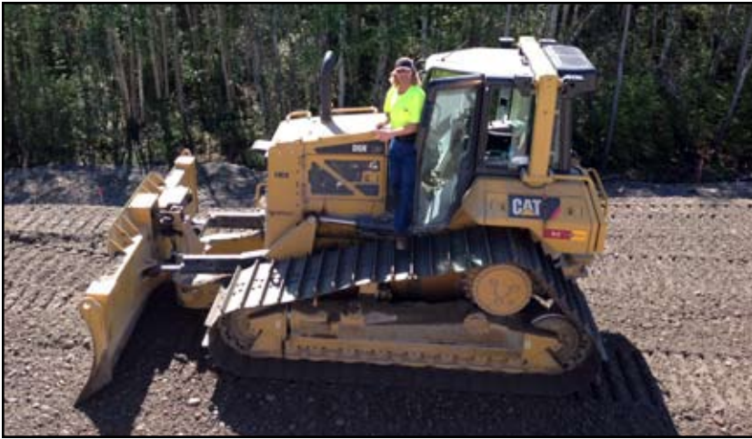
Brian Swarthout- finish dozer operator for HC Contractors in Fairbanks
