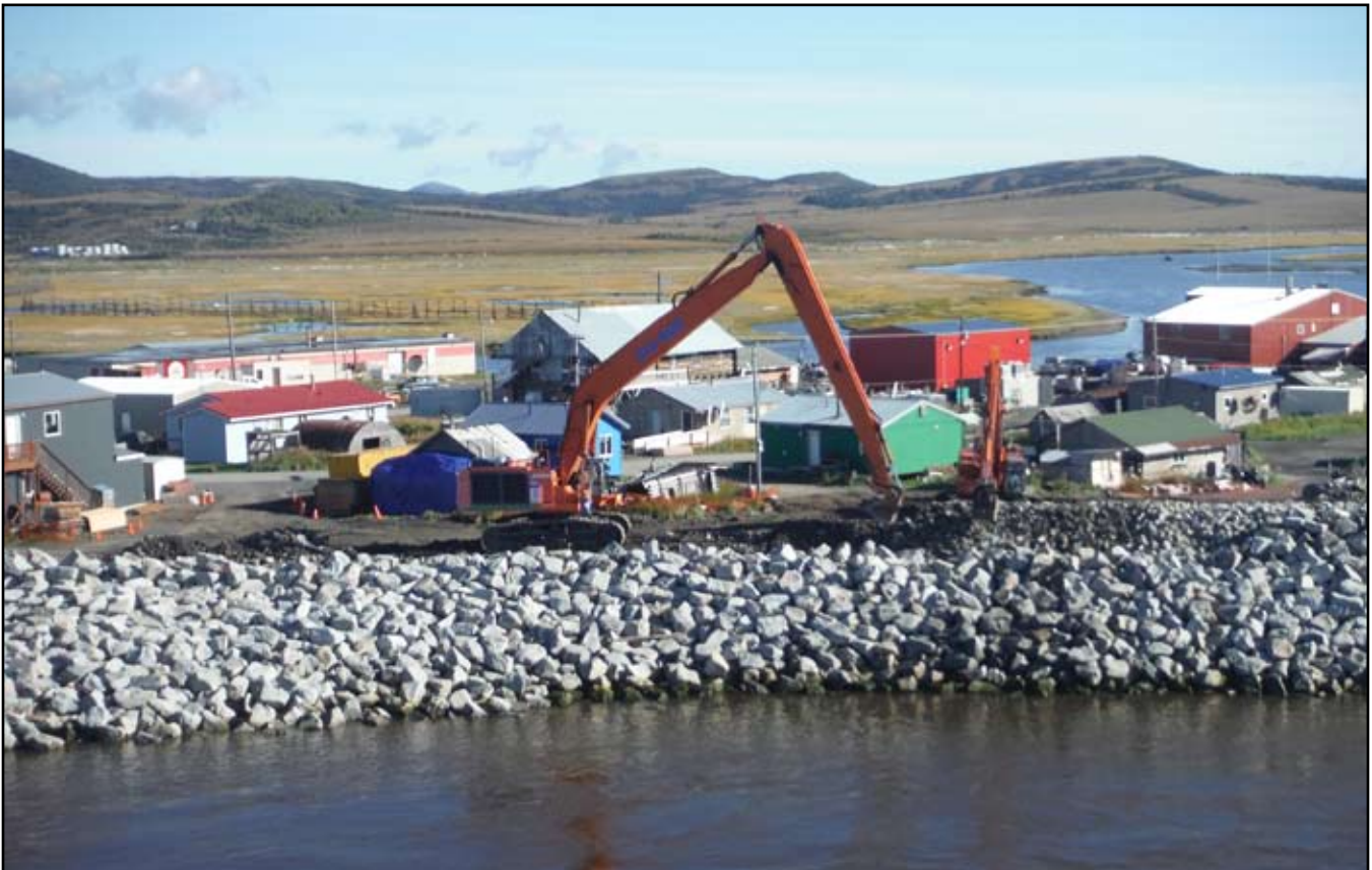
Orion Marine working on the Unalakleet Erosion Control Project
