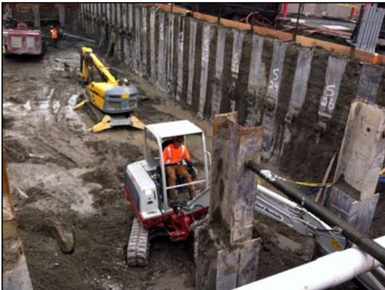
Apprentice Blake Wood on the JCM Northlink project
