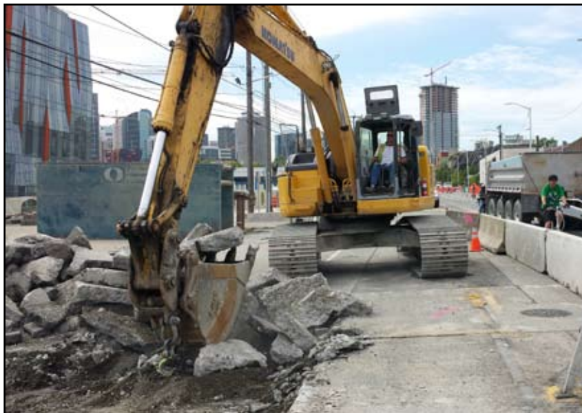
Work continues on the SR99 Tunnel North Access Project
