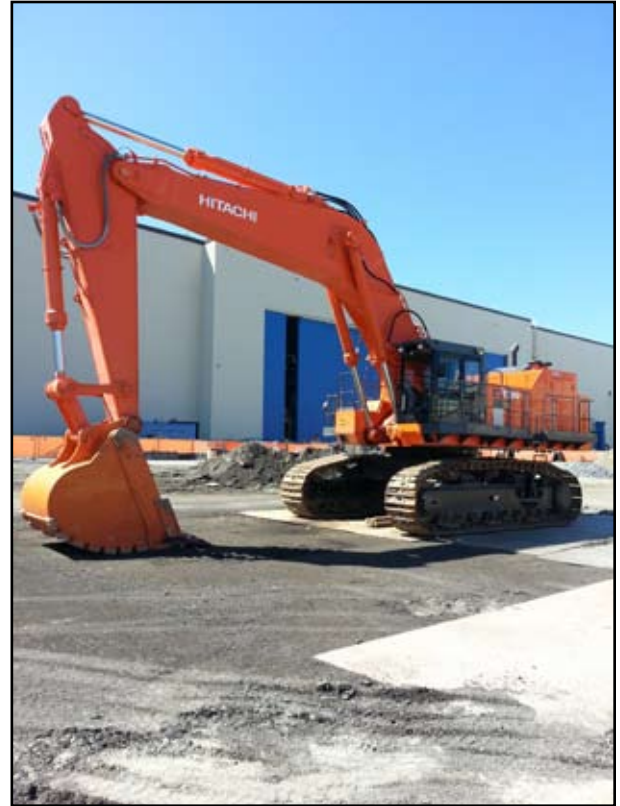
Hitachi 1200 Excavator waiting to start work at the 777x building site.
