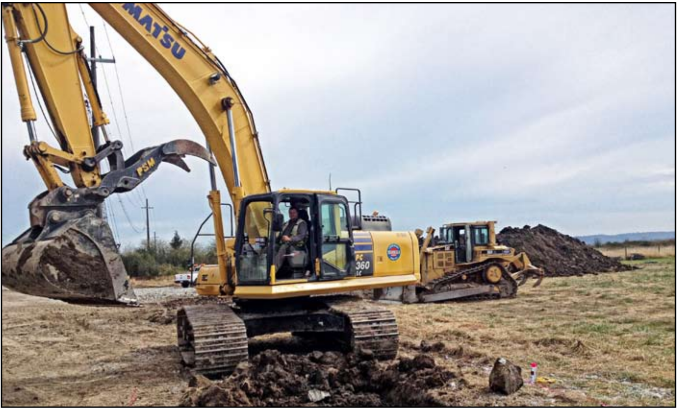
Tony De Marco running the Excavator on a Stanwood project.
