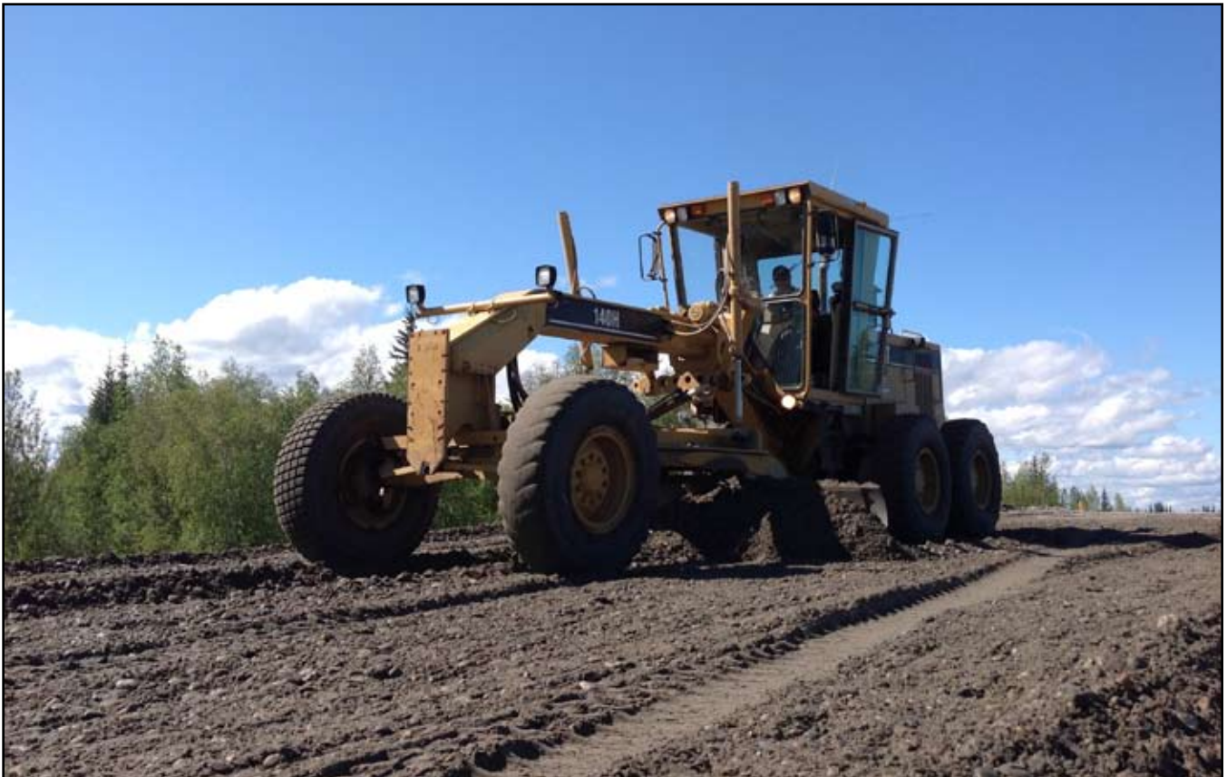
Moose Creek Overpass
